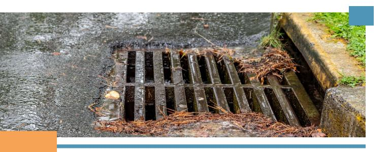
These projects deal with the repair and maintenance of existing storm drains and associated pipelines, as well as the construction of new storm drain infrastructure. Storm drains play an important role in the City and prevent flooding by capturing rainfall and diverting it from our streets to other locations such as retention basins.
