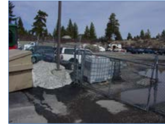
Completely broken up pavement resulting in dirt lot with no drainage.
