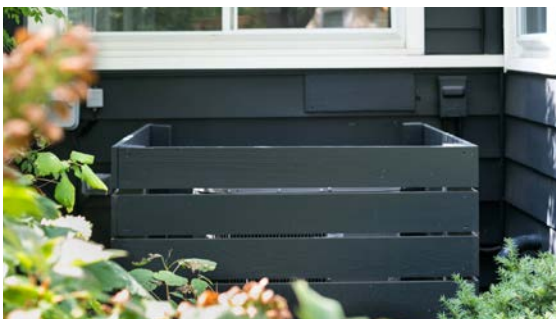
Photo 7.16 - Example of mechanical equipment screen
