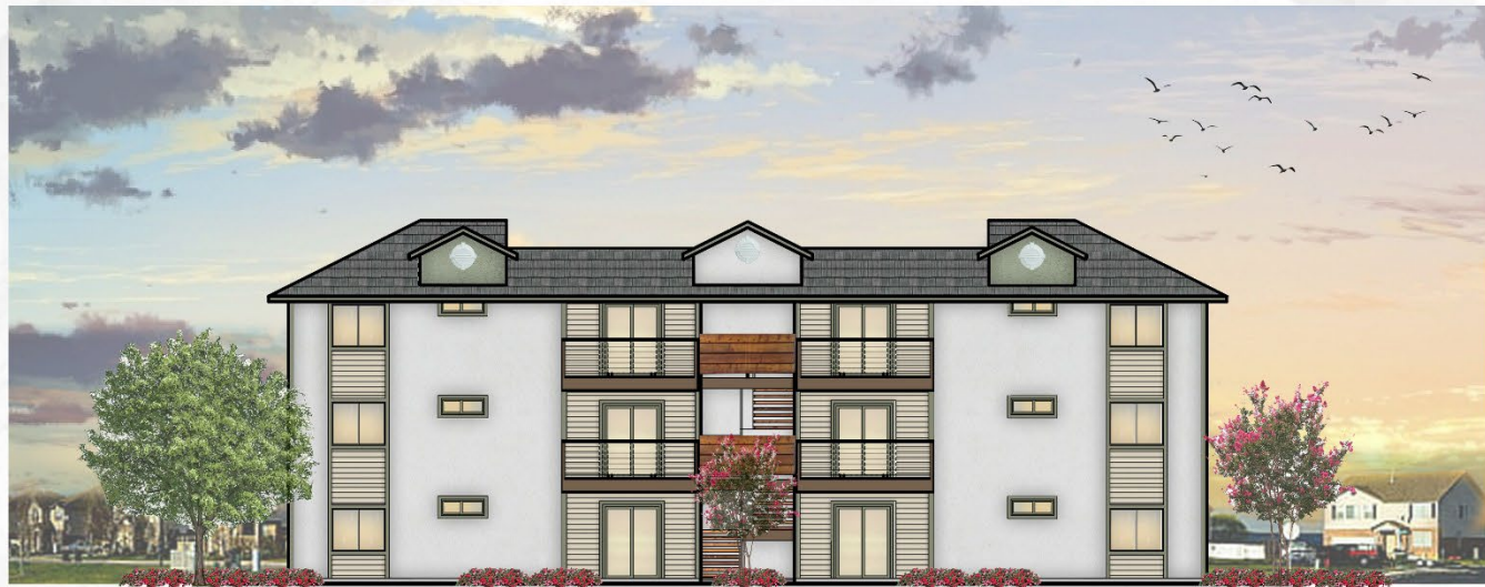
BUILDING "J" (WEST ELEVATION)
