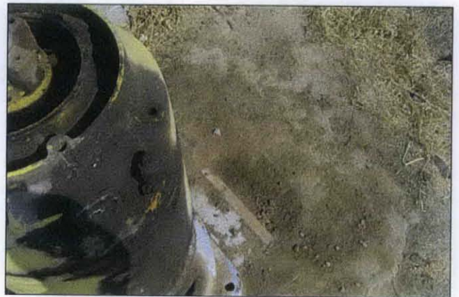
PHOTO 19: Pump motor located on one of well showing signs of hydraulic fluid leak.
