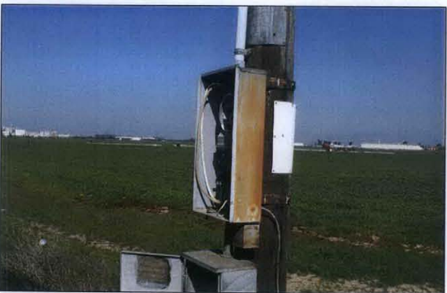
PHOTO 5: Photo showing mounted electrical supply box associated with the well pictured in photo 3.
