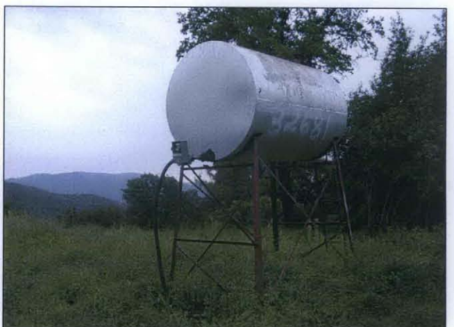
PHOTO 16: Photo showing empty 500-gallon AST located adjacent to the residence shown in Photo 8.
