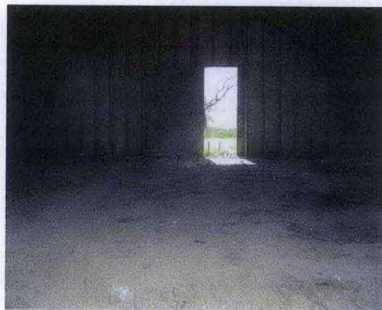
Photo 2: Storage structure from the previous photo showing cement slab and no visible surface cracks in (after clean up).
