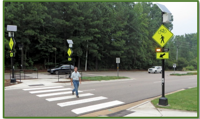
A protected crosswalk with a “RRFB” (Rectangular Rapid Flashing Beacon)
