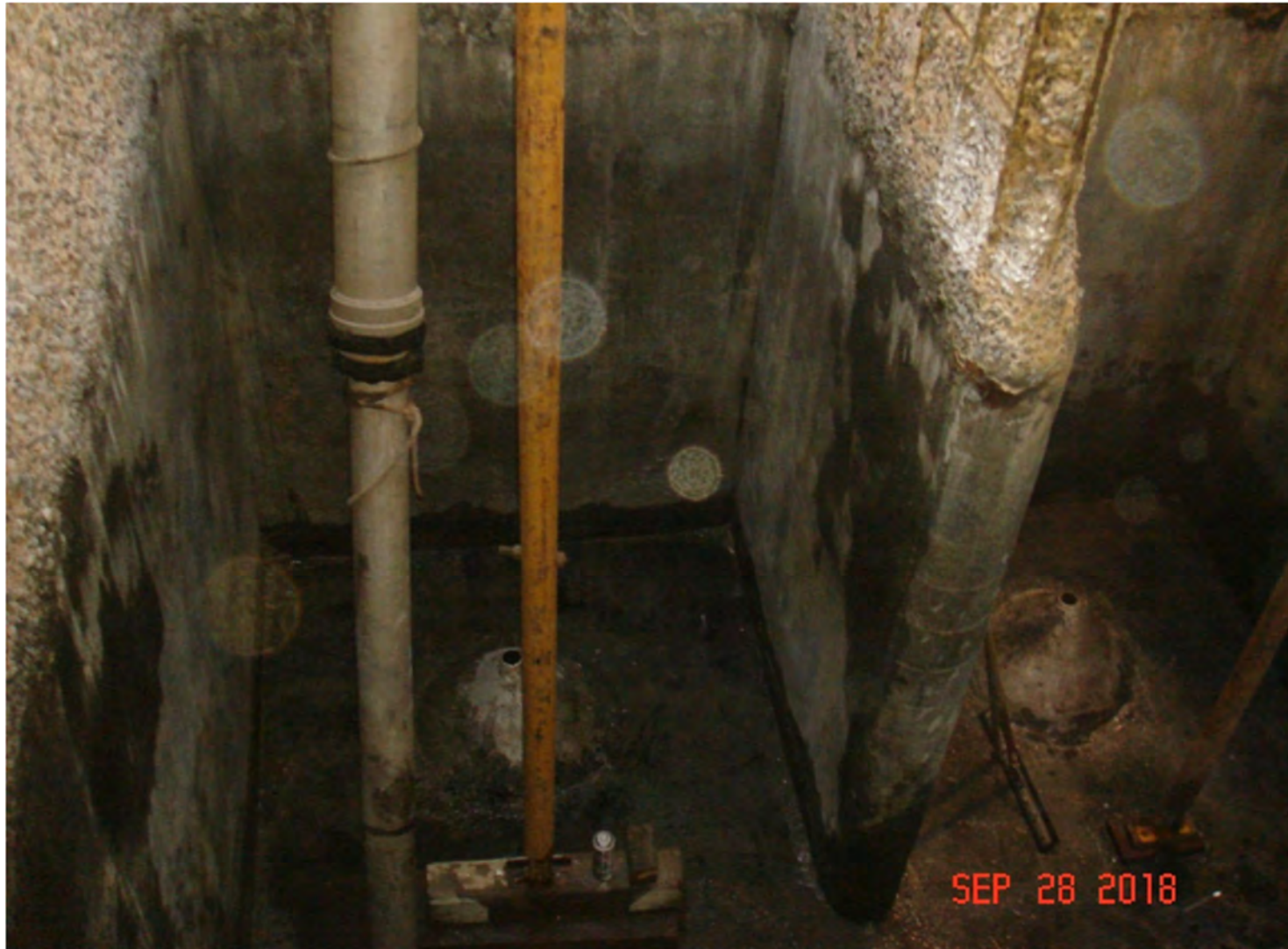
Figure 3 Submerged Concrete Condition: Primary Effluent Pump Station Wetwell
