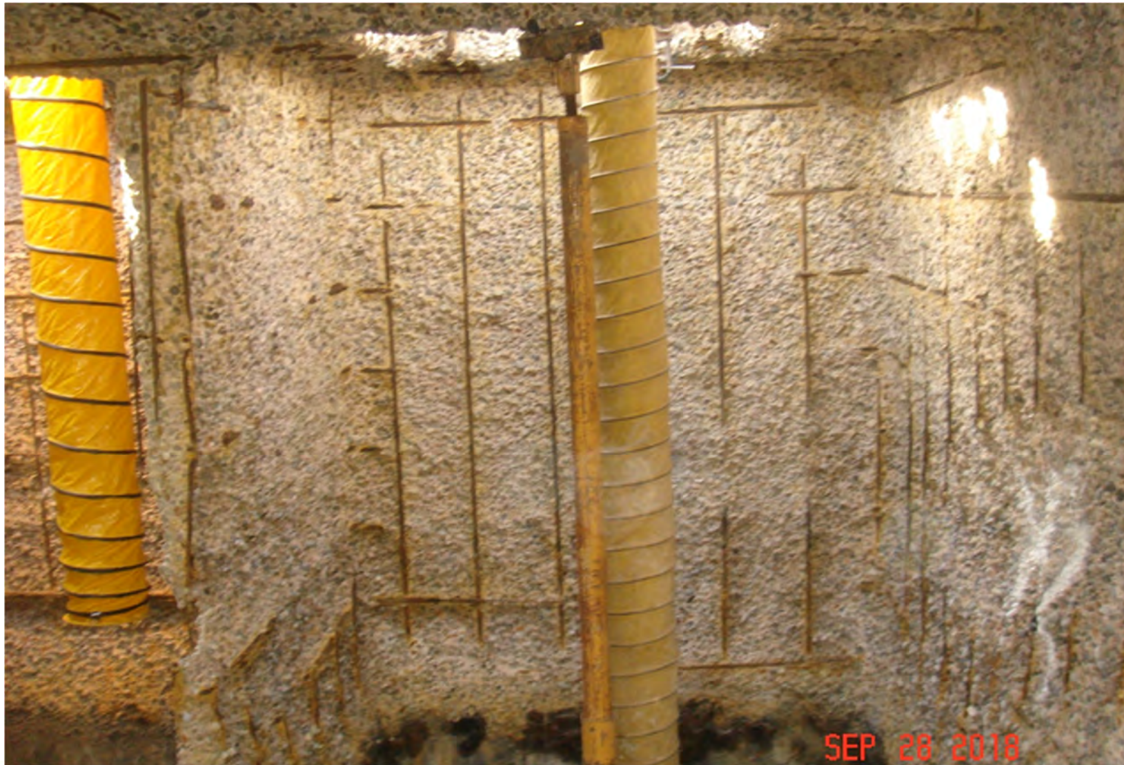
Figure 1 Discovered Condition of Concrete: Primary Effluent Pump Station Wetwell
