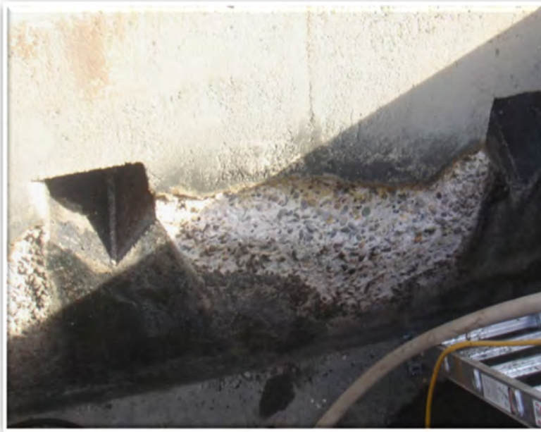
Figure 2 Known Condition of Concrete in Primary Clarifier Channel
