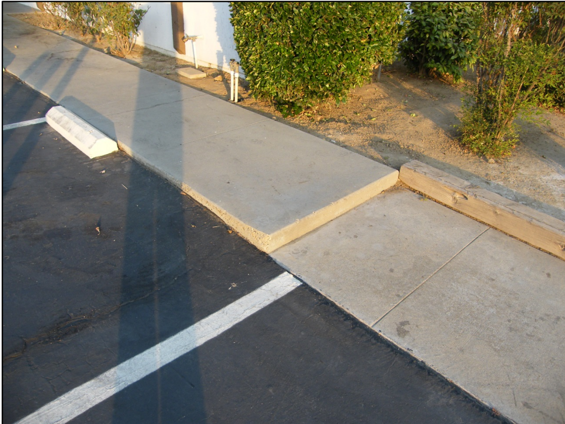
This raised lip will need to be reconstructed into a ramp for the ADA path of travel.
