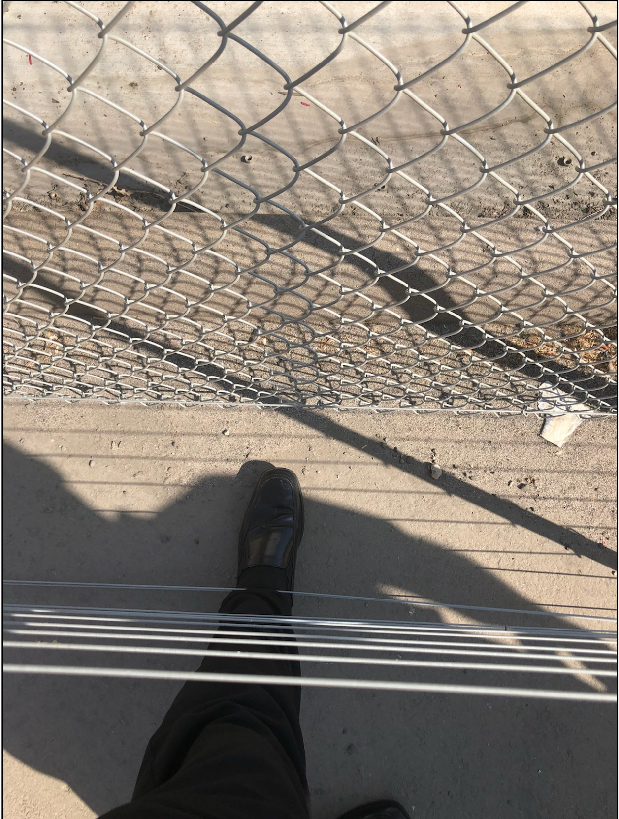
Perception of electrical fence that is 12" away from perimeter fence.
