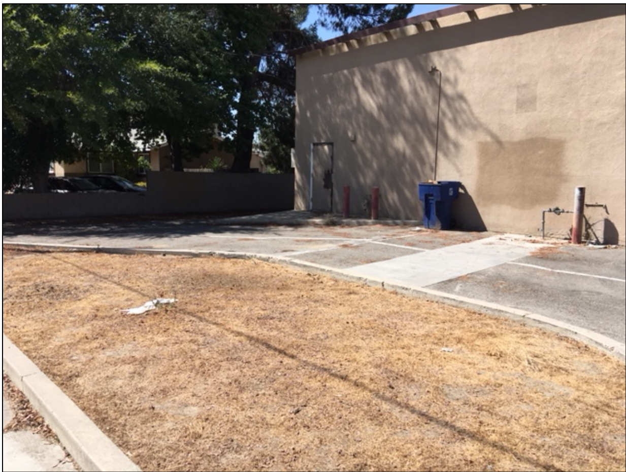
Dead landscaping along the store's right-of-way frontage.
