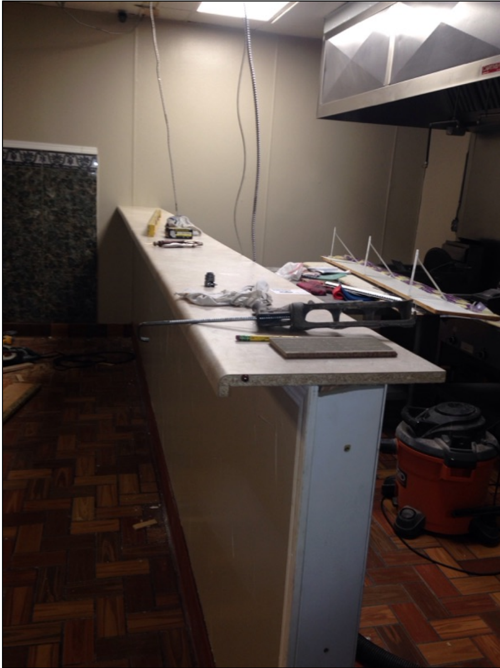
Unpermitted work for reconfiguration of electrical and gas lines.
