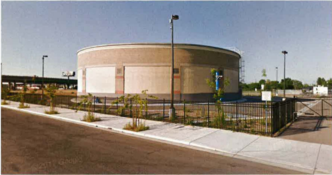
3 million gallon prestressed concrete water storage tank recently constructed for the City of Fresno. City staff had the opportunity to attend a demonstration presented by the contractor/manufacturer of this particular tank.
