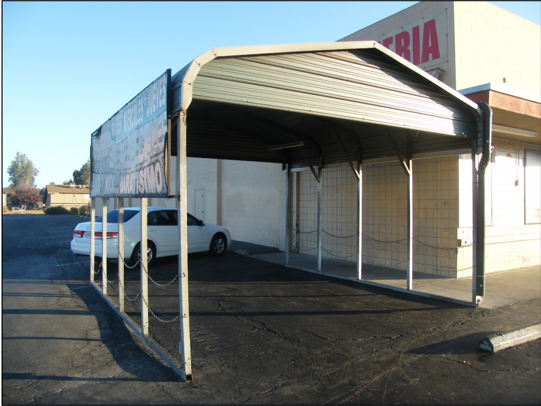
Existing non-permitted carports on the site
