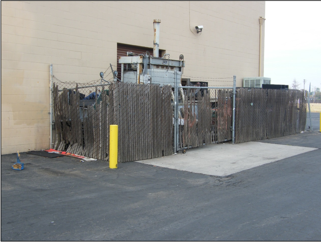
Another storage area on the site
