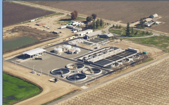
City of Madera Wastewater Treatment Plant
