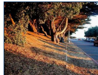
In this photo, a berm (left) is used in place of a wall to block roadway noise.
