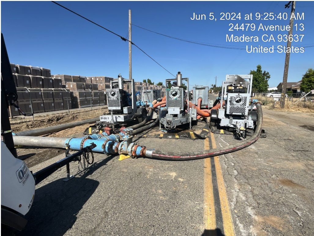
Bypass Pumping Set Up
