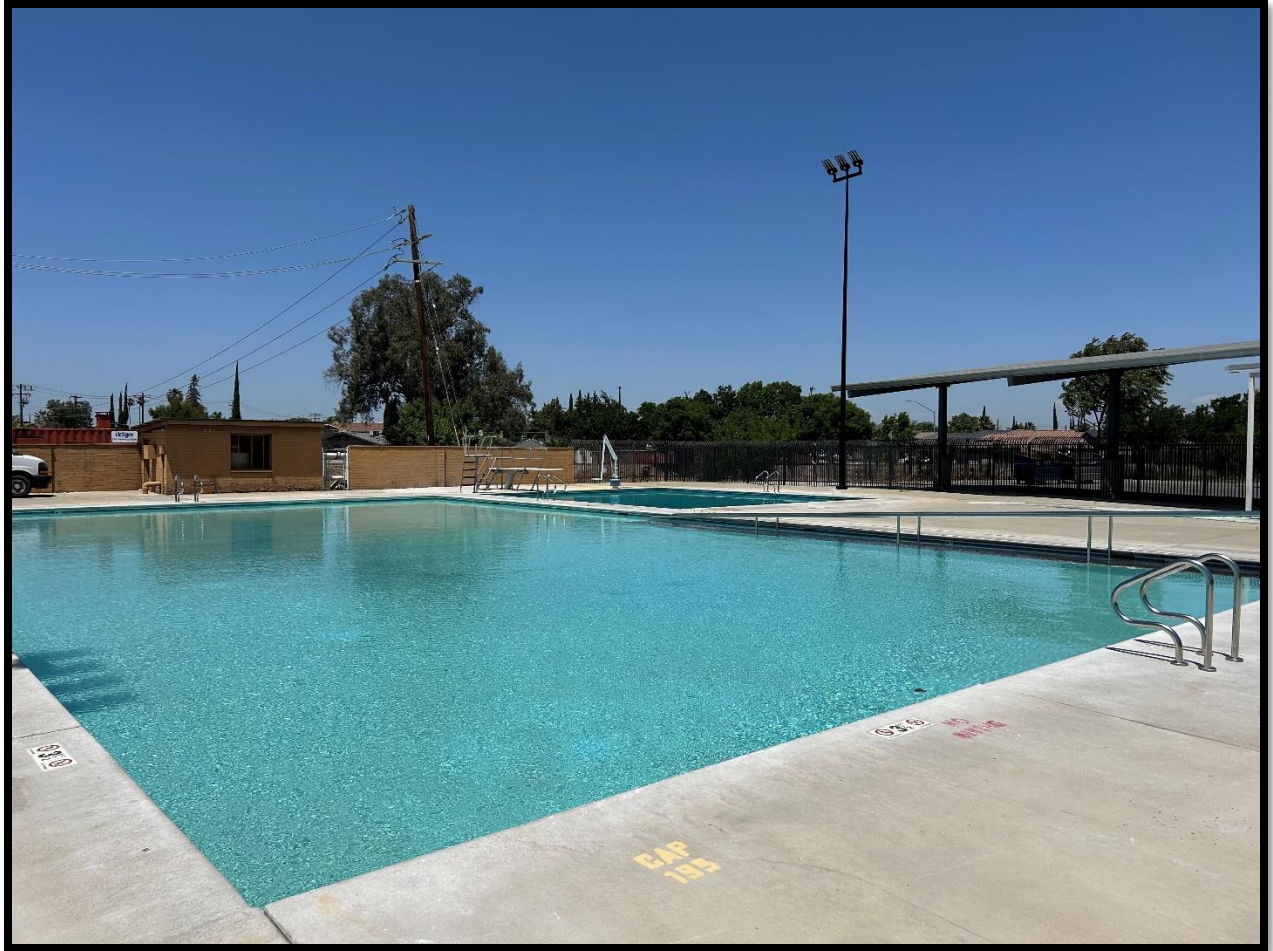
The Image Above Shows the Newly Renovated Lap Pool
