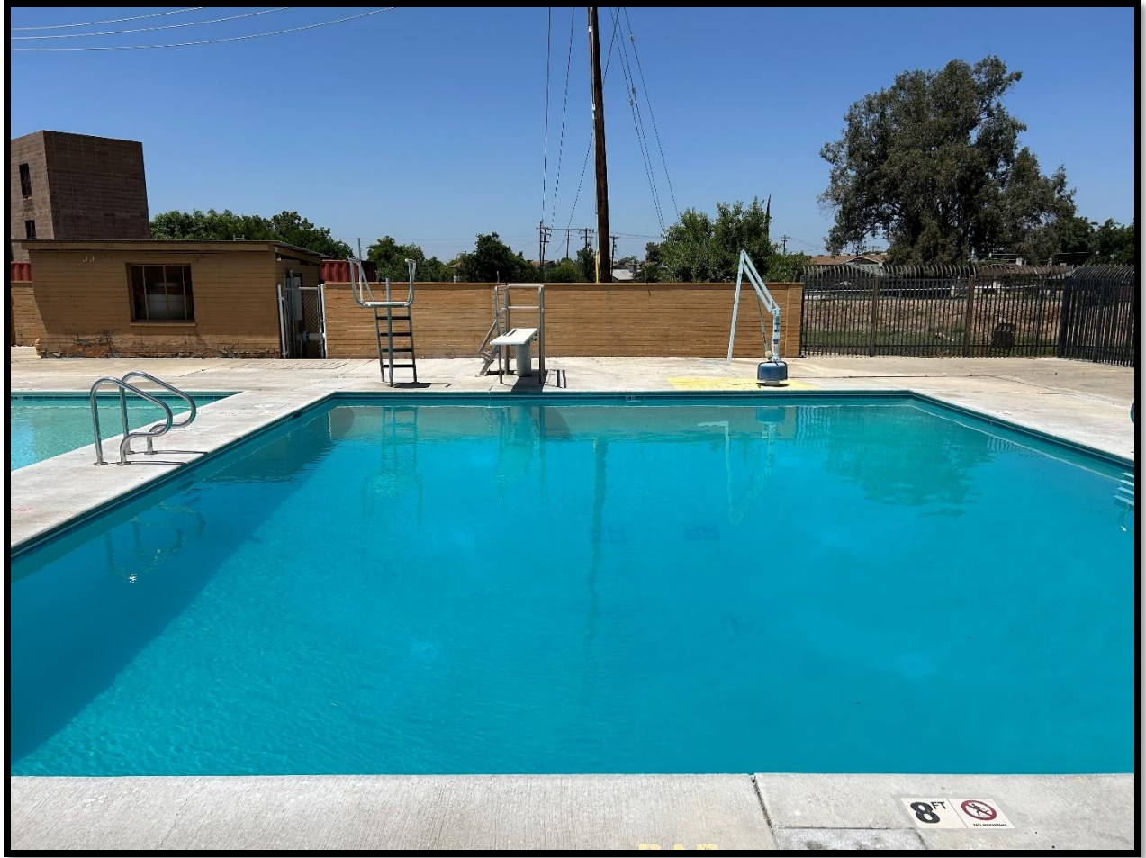
The Image Above Shows the Newly Renovated Dive Pool
