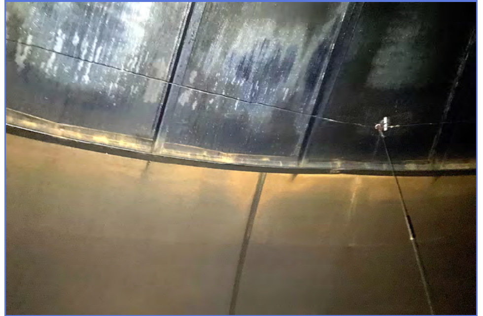
INTERIOR - City of Madera - 1MG Elevated Tank - Maintenance Inspection -009
