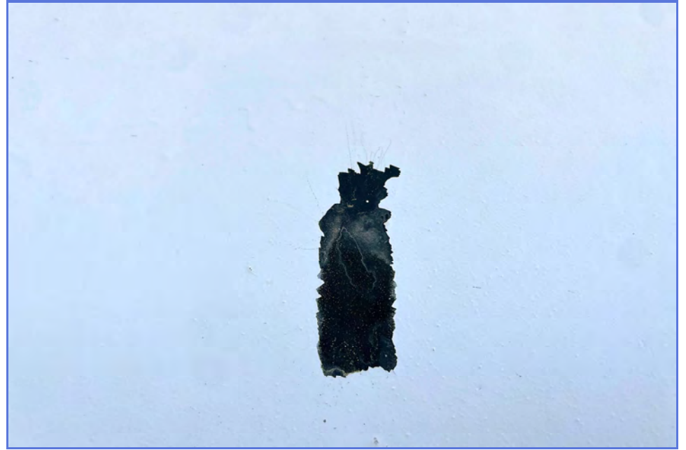
EXTERIOR - City of Madera - 1MG Elevated Tank - Maintenance Inspection -033
