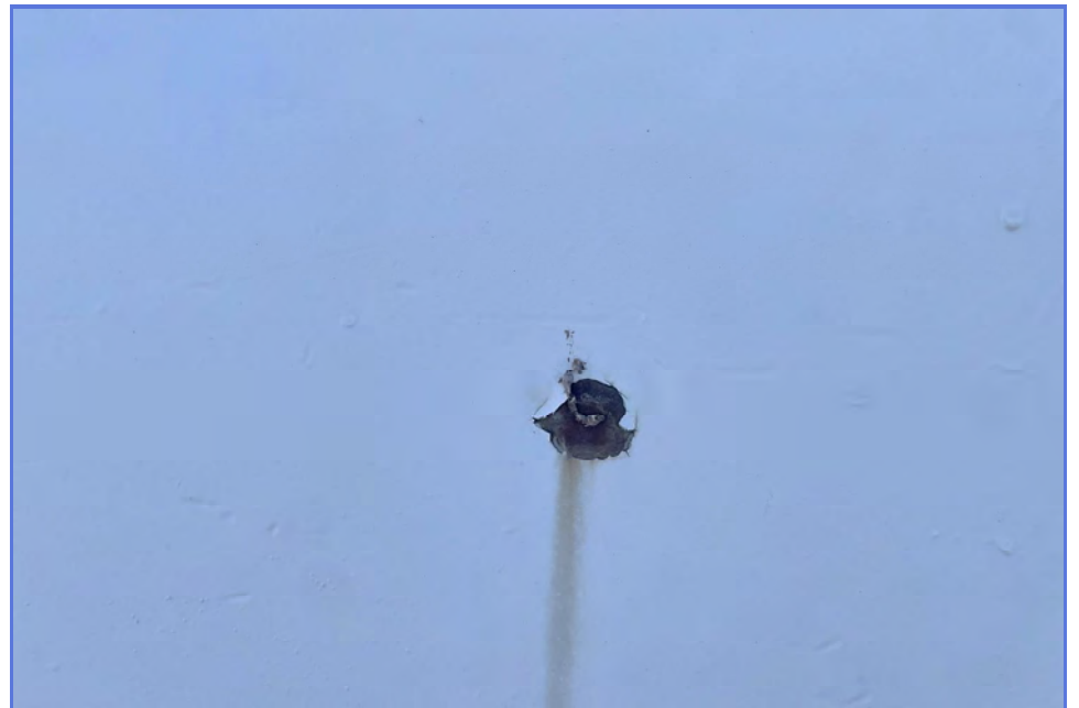
EXTERIOR - City of Madera - 1MG Elevated Tank - Maintenance Inspection -047
