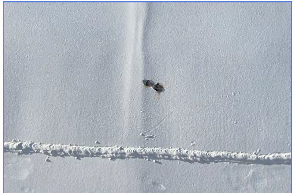
EXTERIOR - City of Madera - 1MG Elevated Tank - Maintenance Inspection -031
