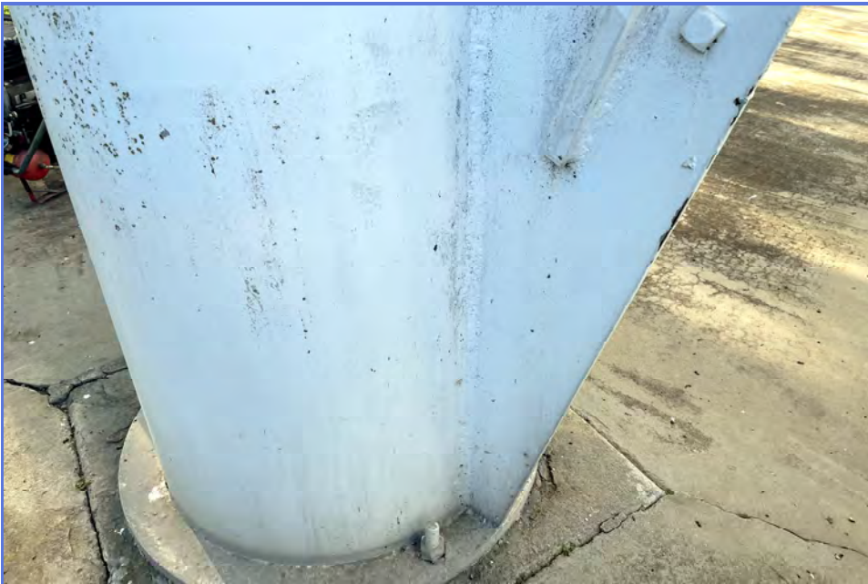
EXTERIOR - City of Madera - 1MG Elevated Tank - Maintenance Inspection -102
