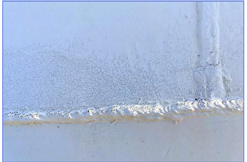
EXTERIOR - City of Madera - 1MG Elevated Tank - Maintenance Inspection -043
