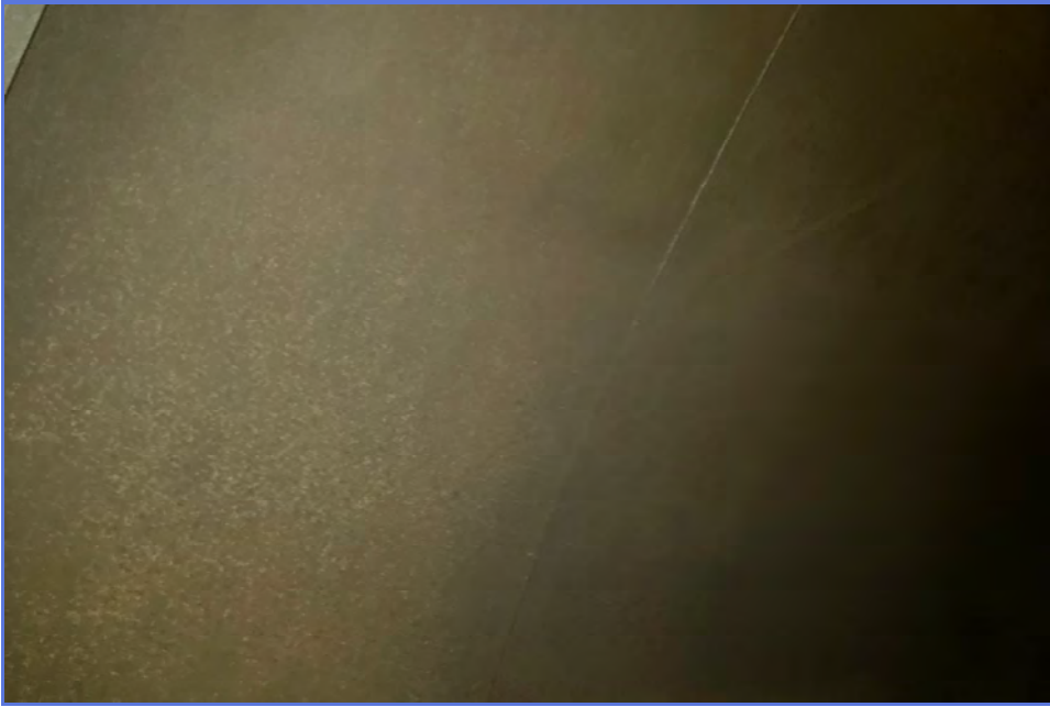
INTERIOR - City of Madera - 1MG Elevated Tank - Maintenance Inspection -016
