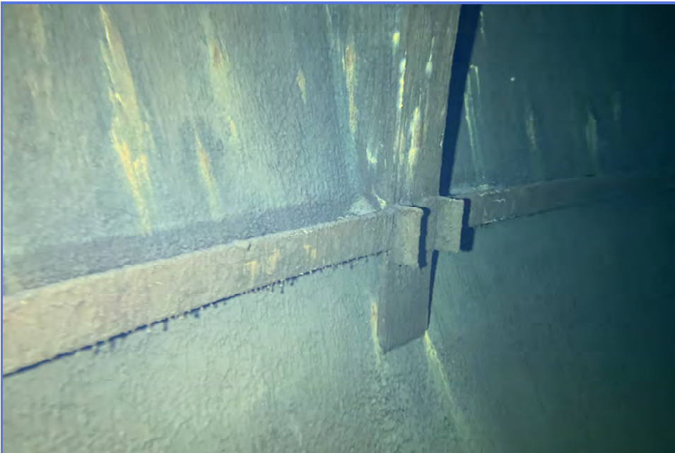
INTERIOR - City of Madera - 1MG Elevated Tank - Maintenance Inspection -038
