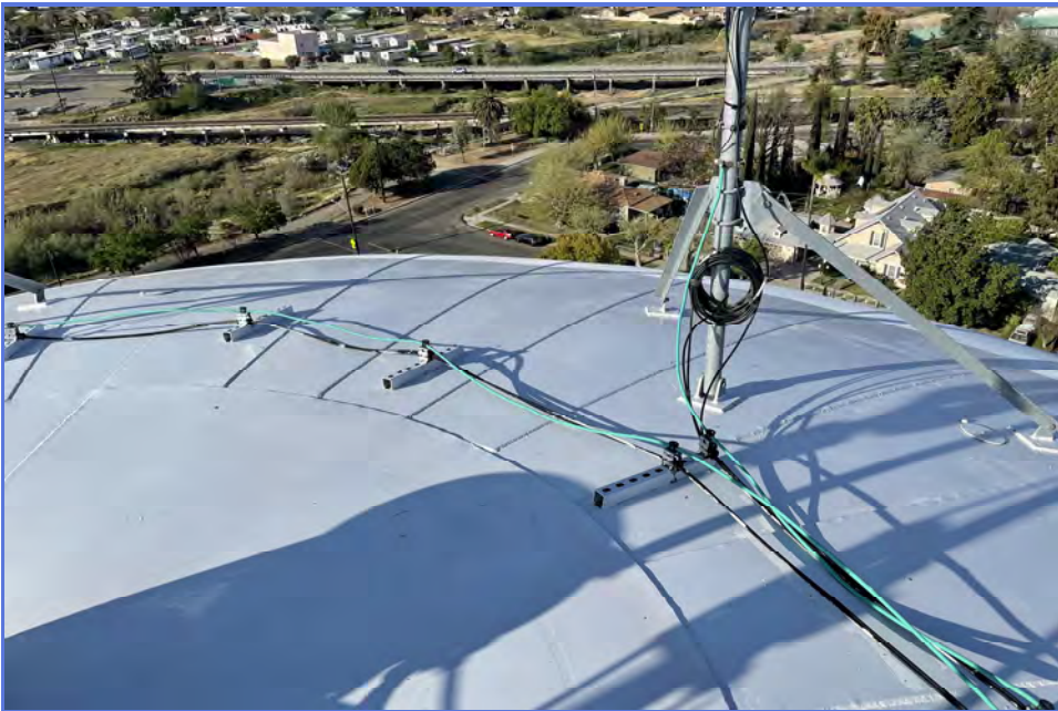
EXTERIOR - City of Madera - 1MG Elevated Tank - Maintenance Inspection -002
