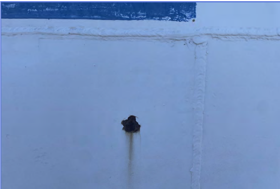
EXTERIOR - City of Madera - 1MG Elevated Tank - Maintenance Inspection -010
