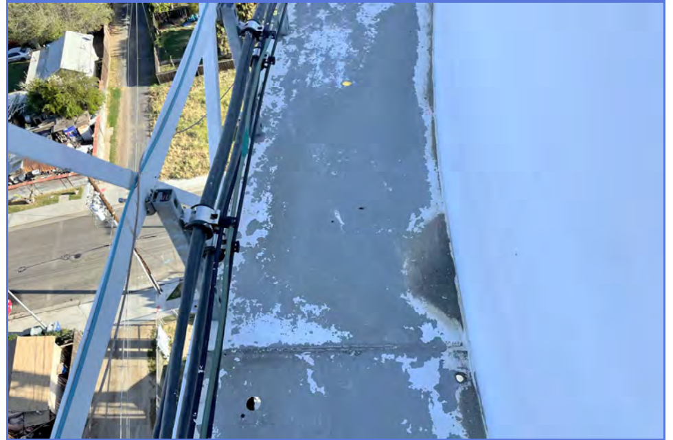
EXTERIOR - City of Madera - 1MG Elevated Tank - Maintenance Inspection -053
