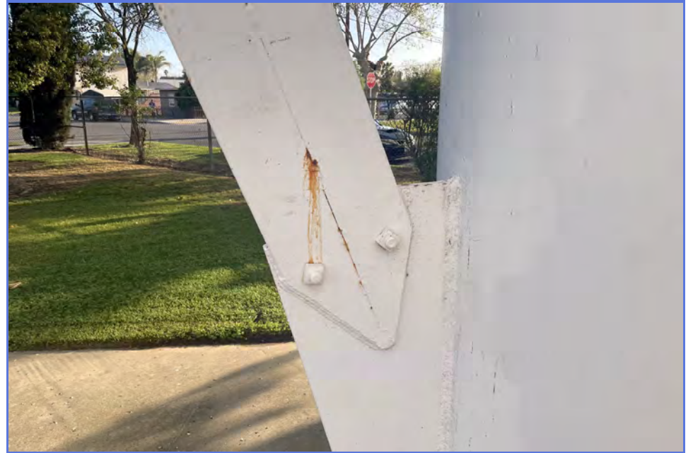
EXTERIOR - City of Madera - 1MG Elevated Tank - Maintenance Inspection -101
