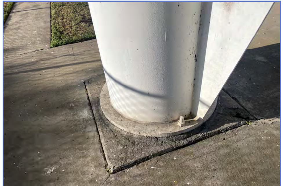
EXTERIOR - City of Madera - 1MG Elevated Tank - Maintenance Inspection -091
