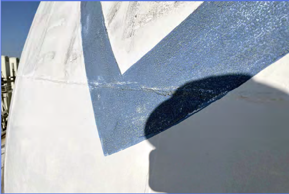
EXTERIOR - City of Madera - 1MG Elevated Tank - Maintenance Inspection -028
