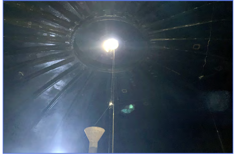
INTERIOR - City of Madera - 1MG Elevated Tank - Maintenance Inspection -001
