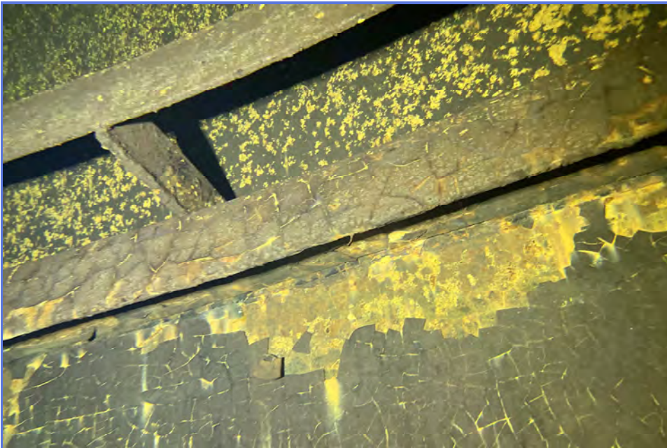
INTERIOR - City of Madera - 1MG Elevated Tank - Maintenance Inspection -034
