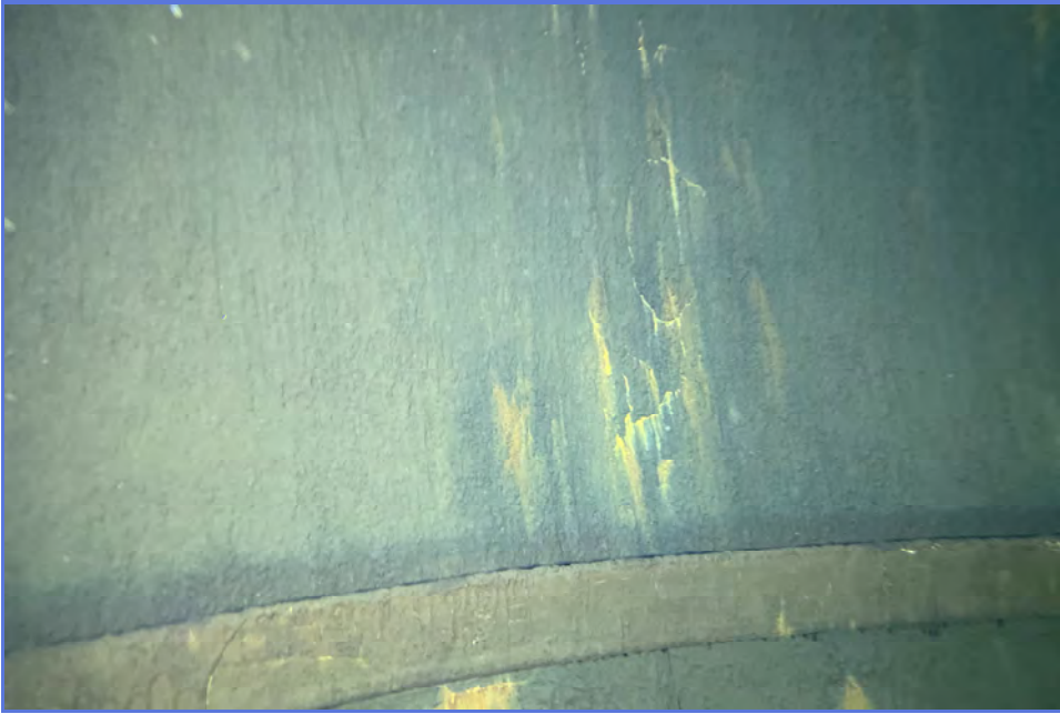
INTERIOR - City of Madera - 1MG Elevated Tank - Maintenance Inspection -044
