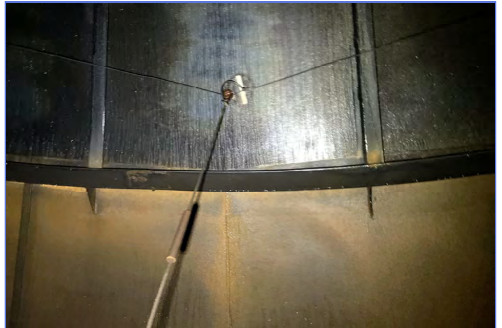
INTERIOR - City of Madera - 1MG Elevated Tank - Maintenance Inspection -011
