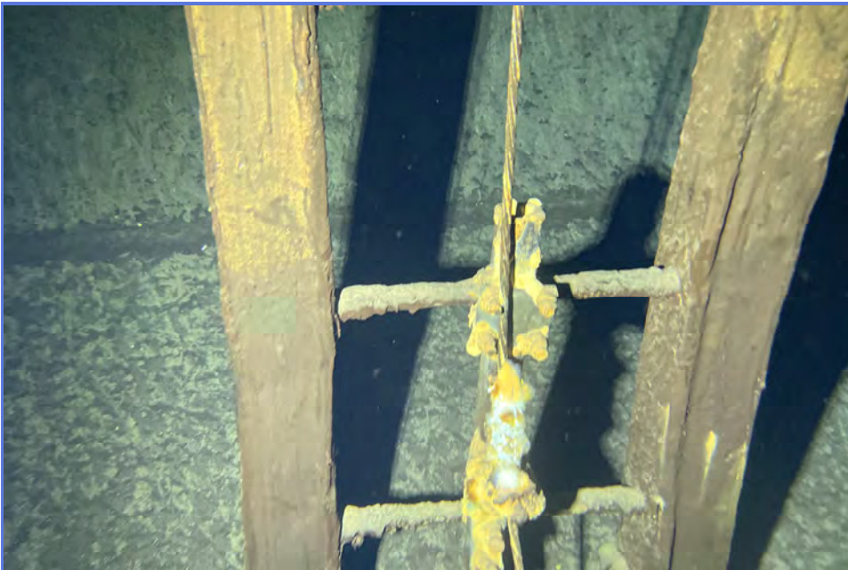
INTERIOR - City of Madera - 1MG Elevated Tank - Maintenance Inspection -074
