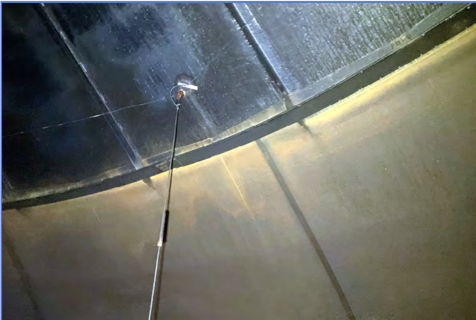
INTERIOR - City of Madera - 1MG Elevated Tank - Maintenance Inspection -010
