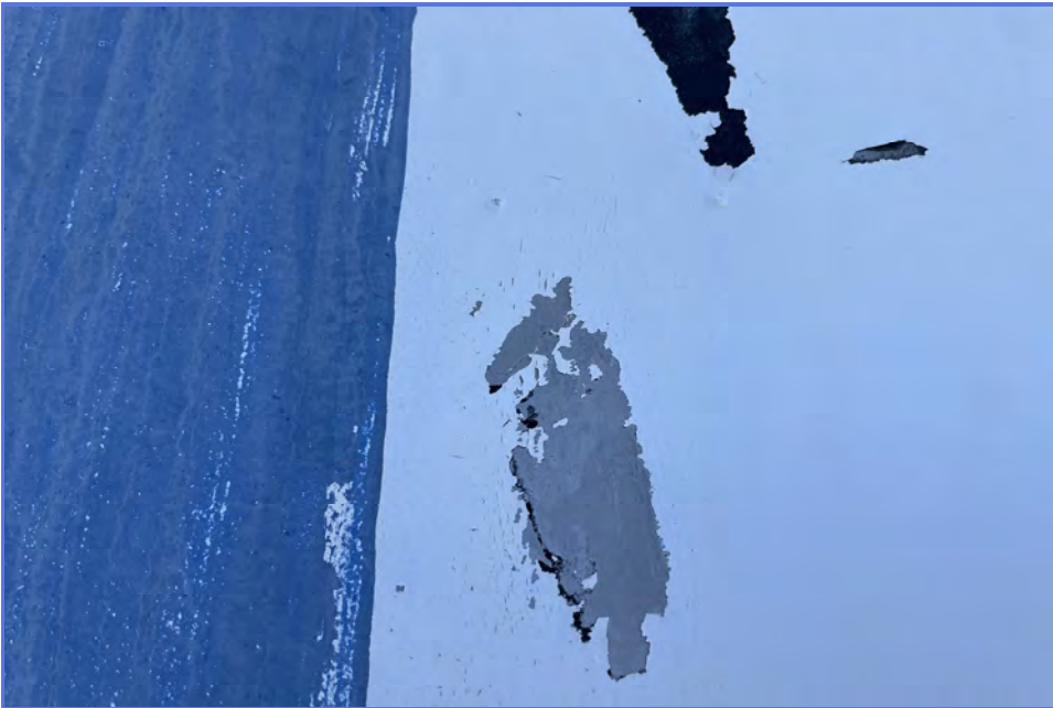
EXTERIOR - City of Madera - 1MG Elevated Tank - Maintenance Inspection -014
