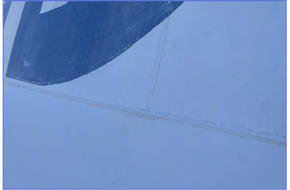
EXTERIOR - City of Madera - 1MG Elevated Tank - Maintenance Inspection -021
