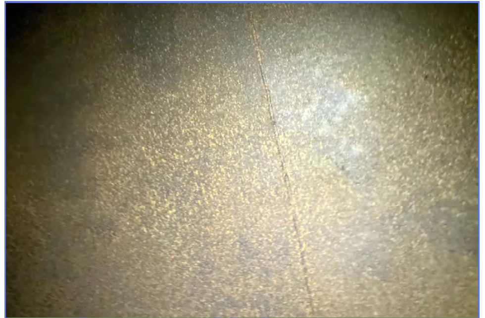
INTERIOR - City of Madera - 1MG Elevated Tank - Maintenance Inspection -019
