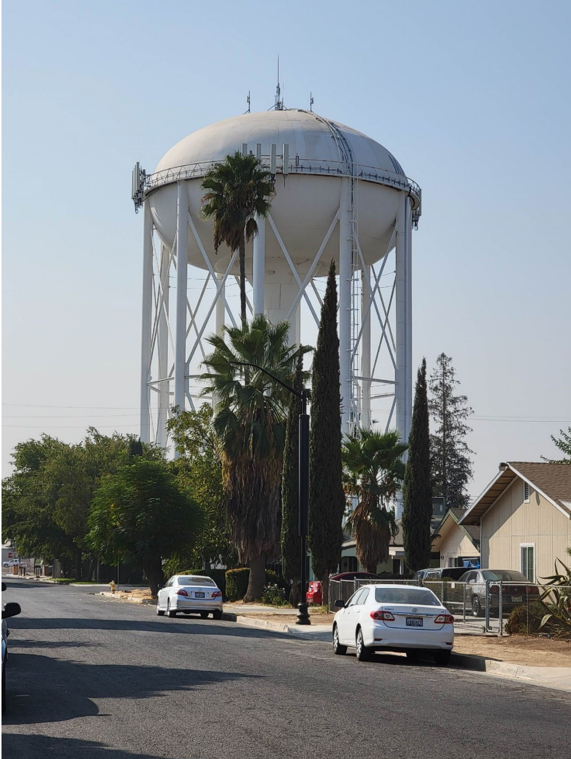
Figure 3-1: Loy E Cook Water Tower Photograph
