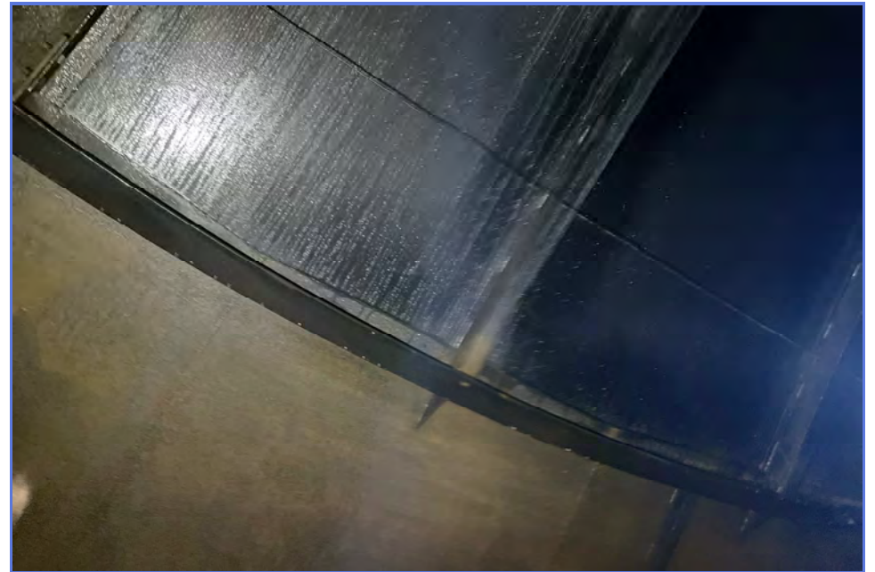
INTERIOR - City of Madera - 1MG Elevated Tank - Maintenance Inspection -003
