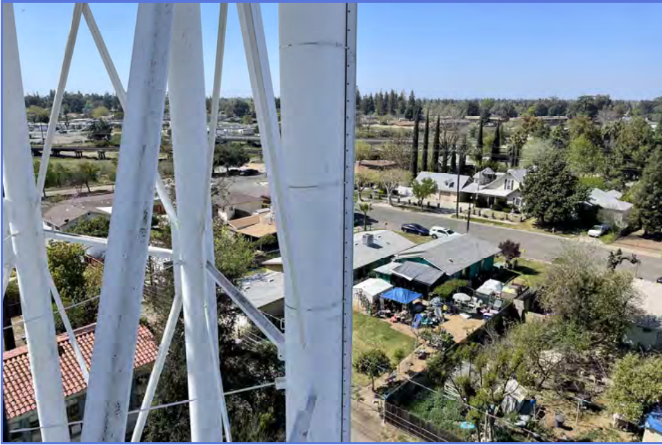
EXTERIOR - City of Madera - 1MG Elevated Tank - Maintenance Inspection -076
