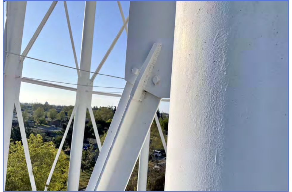
EXTERIOR - City of Madera - 1MG Elevated Tank - Maintenance Inspection -077
