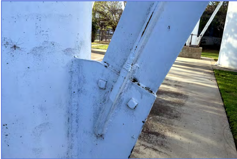
EXTERIOR - City of Madera - 1MG Elevated Tank - Maintenance Inspection -096
