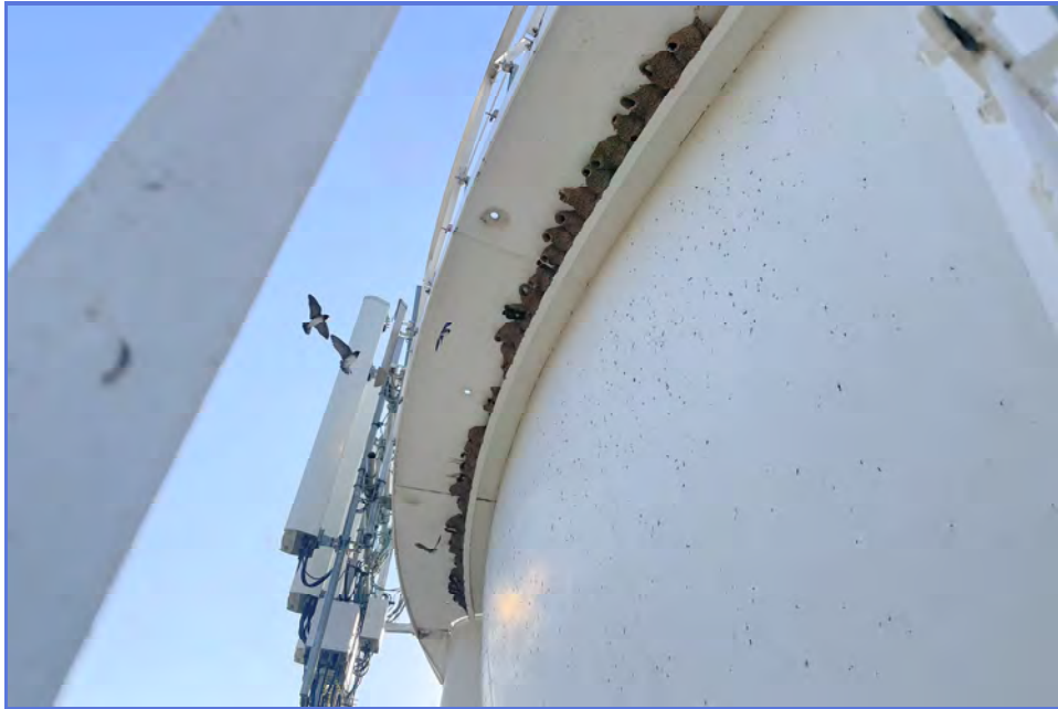
EXTERIOR - City of Madera - 1MG Elevated Tank - Maintenance Inspection -068
