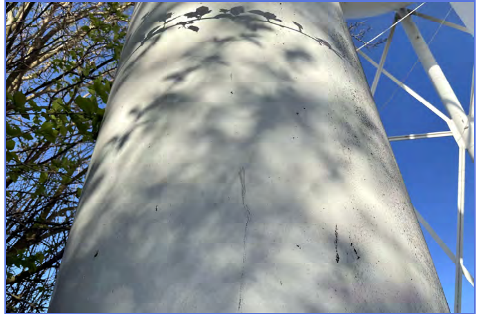
EXTERIOR - City of Madera - 1MG Elevated Tank - Maintenance Inspection -089
