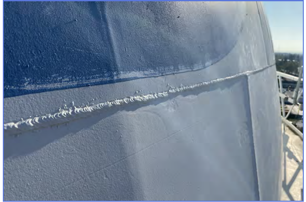
EXTERIOR - City of Madera - 1MG Elevated Tank - Maintenance Inspection -013
