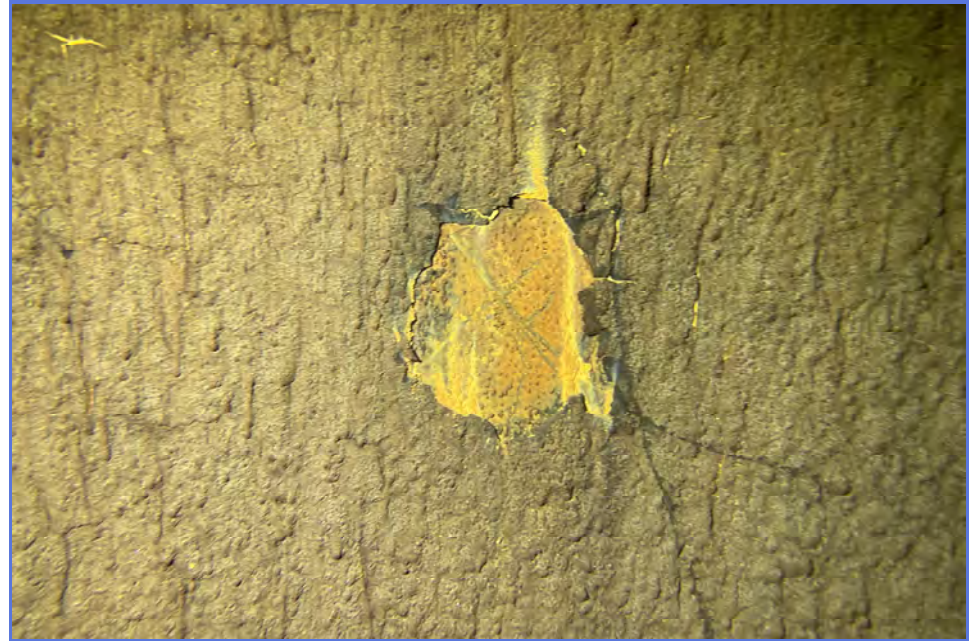
INTERIOR - City of Madera - 1MG Elevated Tank - Maintenance Inspection -049
