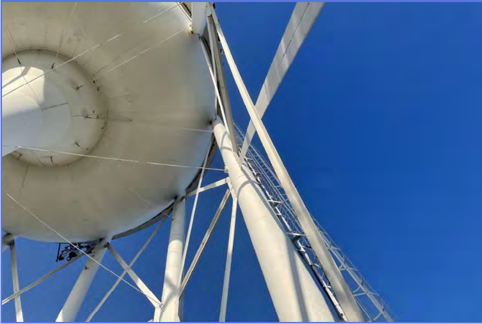
EXTERIOR - City of Madera - 1MG Elevated Tank - Maintenance Inspection -072
