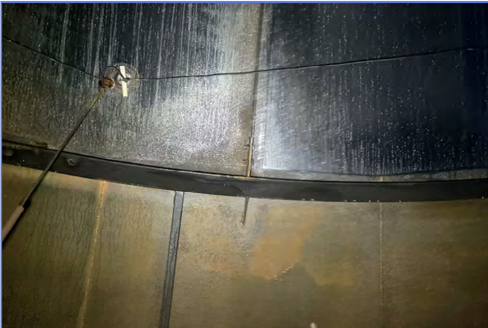
INTERIOR - City of Madera - 1MG Elevated Tank - Maintenance Inspection -014
