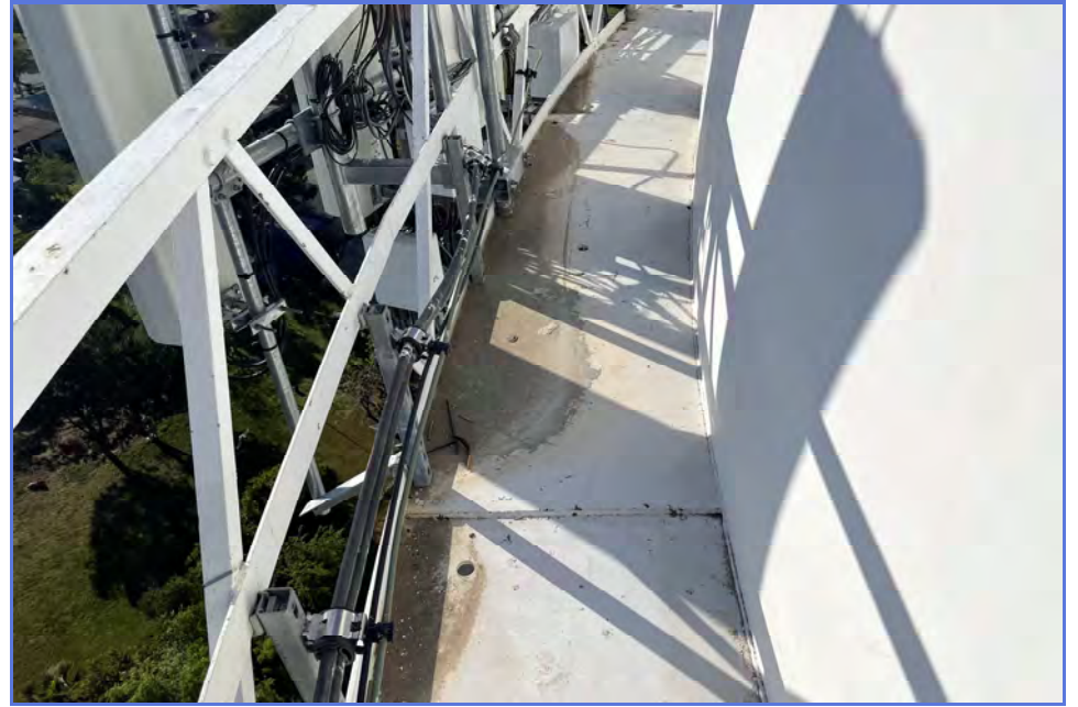
EXTERIOR - City of Madera - 1MG Elevated Tank - Maintenance Inspection -061
