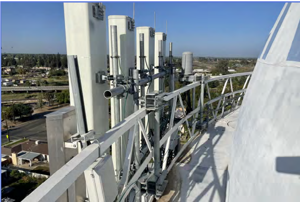
EXTERIOR - City of Madera - 1MG Elevated Tank - Maintenance Inspection -058
