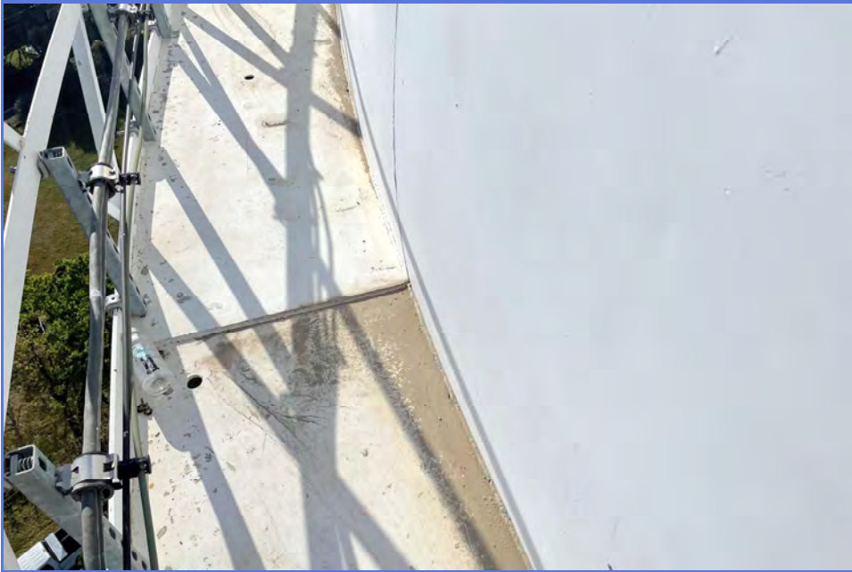
EXTERIOR - City of Madera - 1MG Elevated Tank - Maintenance Inspection -052
