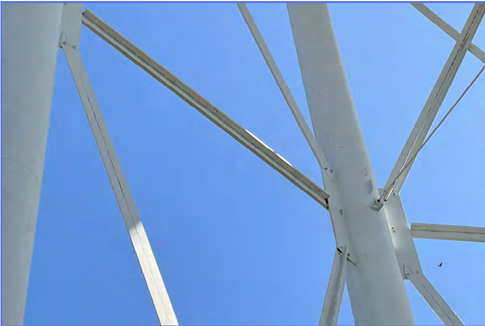
EXTERIOR - City of Madera - 1MG Elevated Tank - Maintenance Inspection -078
