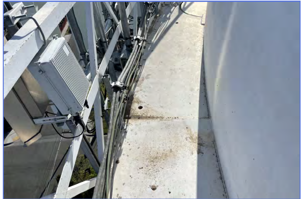
EXTERIOR - City of Madera - 1MG Elevated Tank - Maintenance Inspection -063
