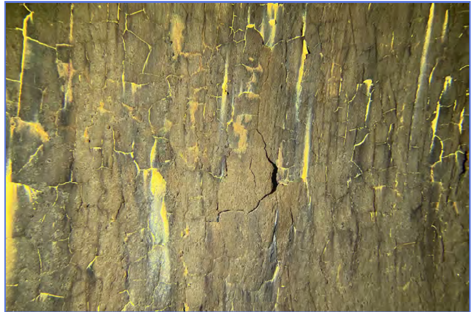
INTERIOR - City of Madera - 1MG Elevated Tank - Maintenance Inspection -055
