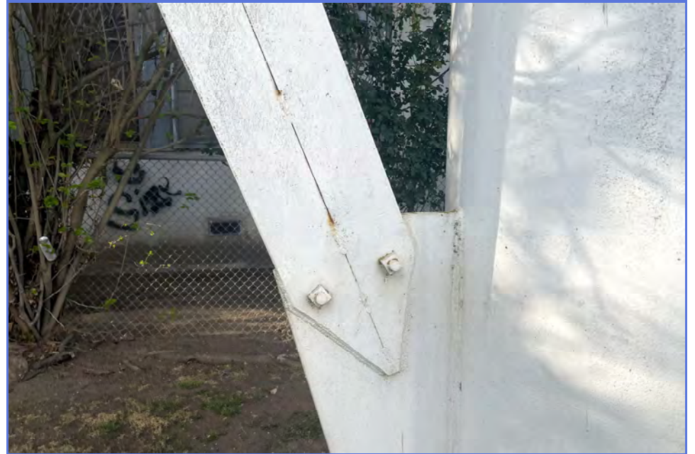
EXTERIOR - City of Madera - 1MG Elevated Tank - Maintenance Inspection -095
