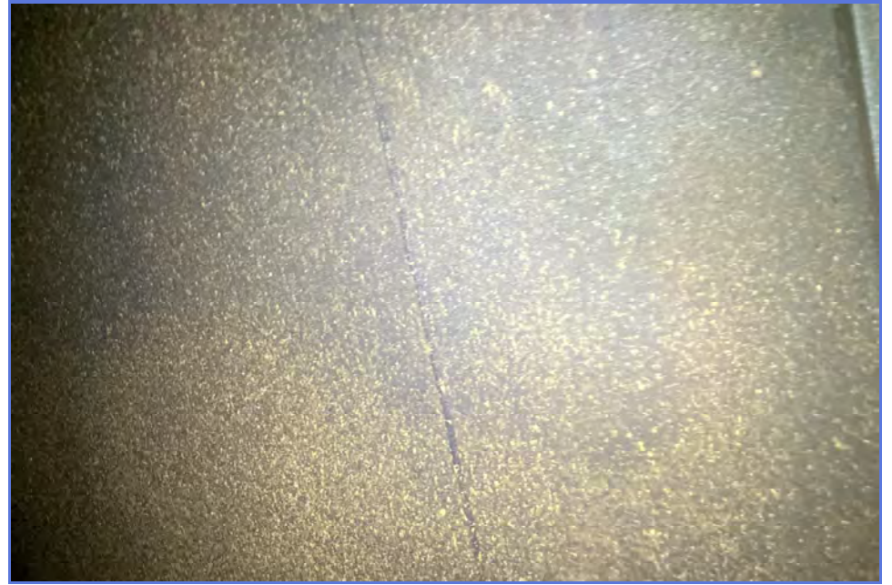
INTERIOR - City of Madera - 1MG Elevated Tank - Maintenance Inspection -017
