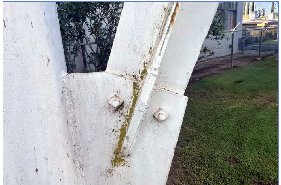
EXTERIOR - City of Madera - 1MG Elevated Tank - Maintenance Inspection -099
