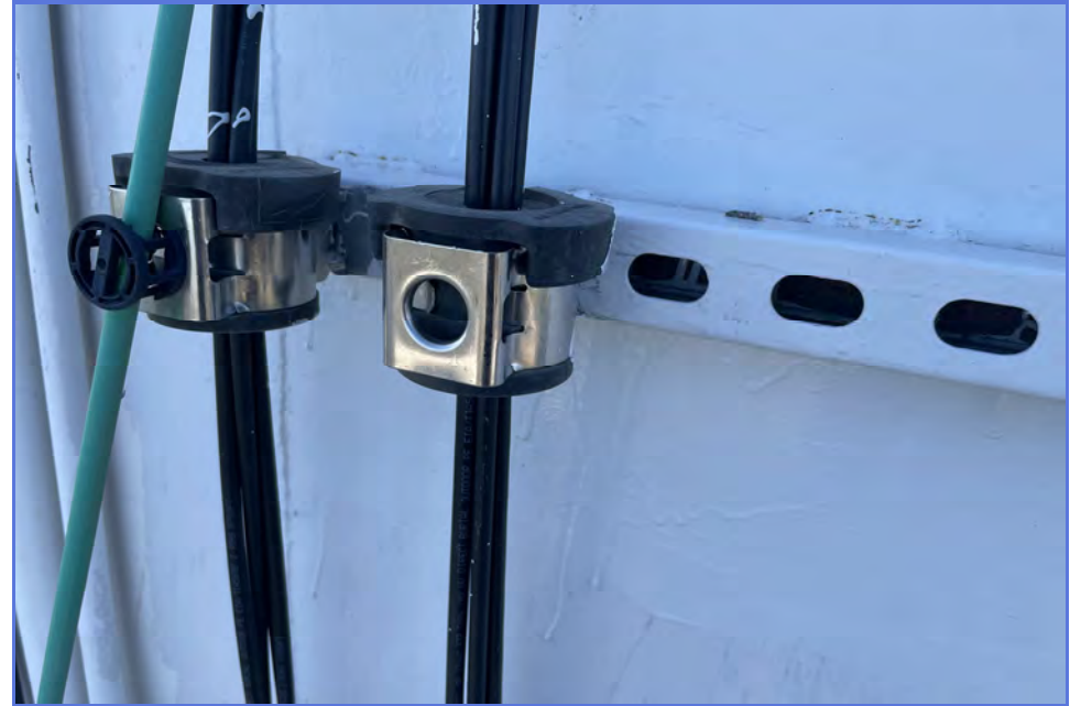
EXTERIOR - City of Madera - 1MG Elevated Tank - Maintenance Inspection -009
