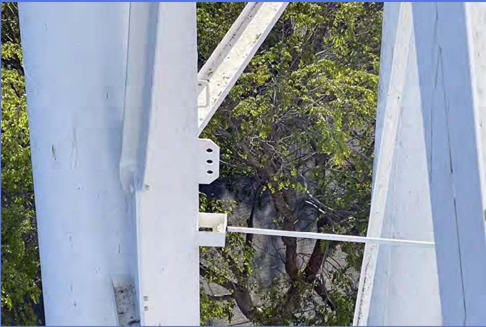
EXTERIOR - City of Madera - 1MG Elevated Tank - Maintenance Inspection -080
