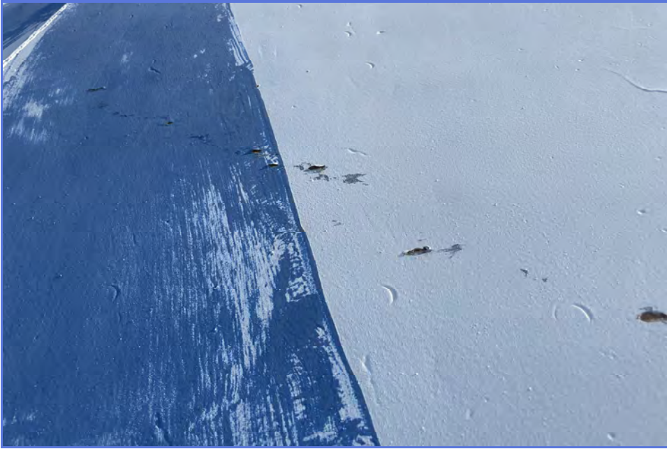
EXTERIOR - City of Madera - 1MG Elevated Tank - Maintenance Inspection -012
