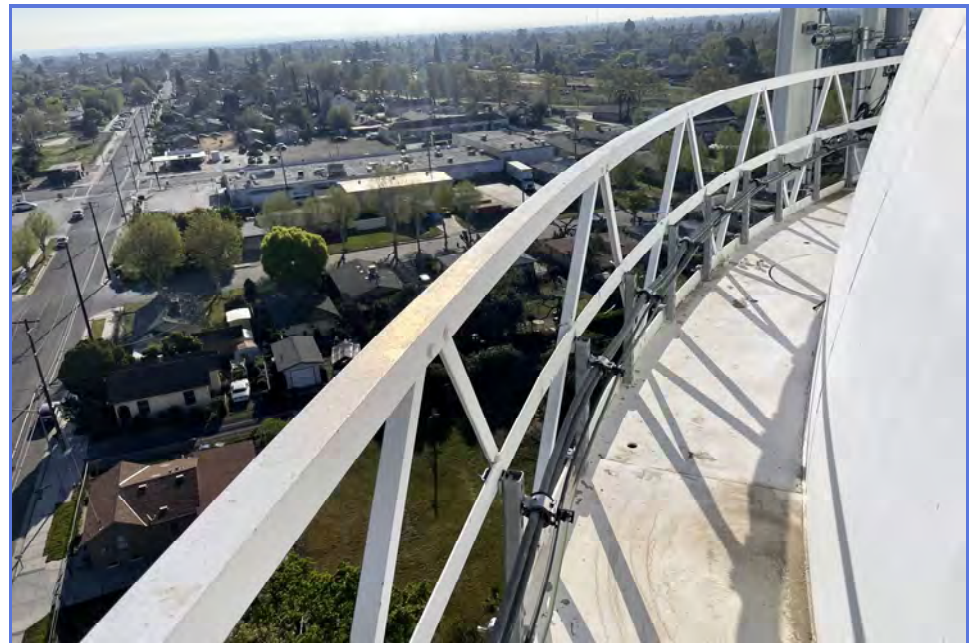
EXTERIOR - City of Madera - 1MG Elevated Tank - Maintenance Inspection -059
