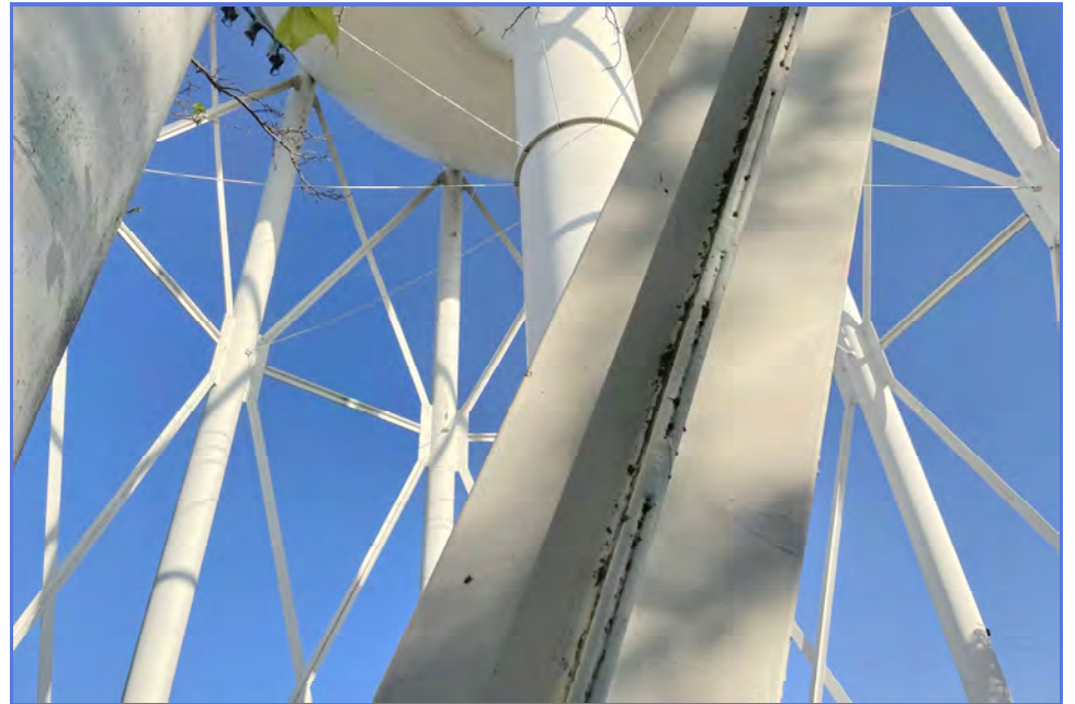
EXTERIOR - City of Madera - 1MG Elevated Tank - Maintenance Inspection -083
