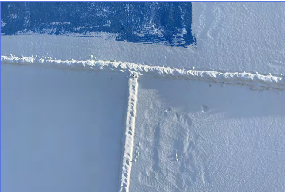
EXTERIOR - City of Madera - 1MG Elevated Tank - Maintenance Inspection -026
