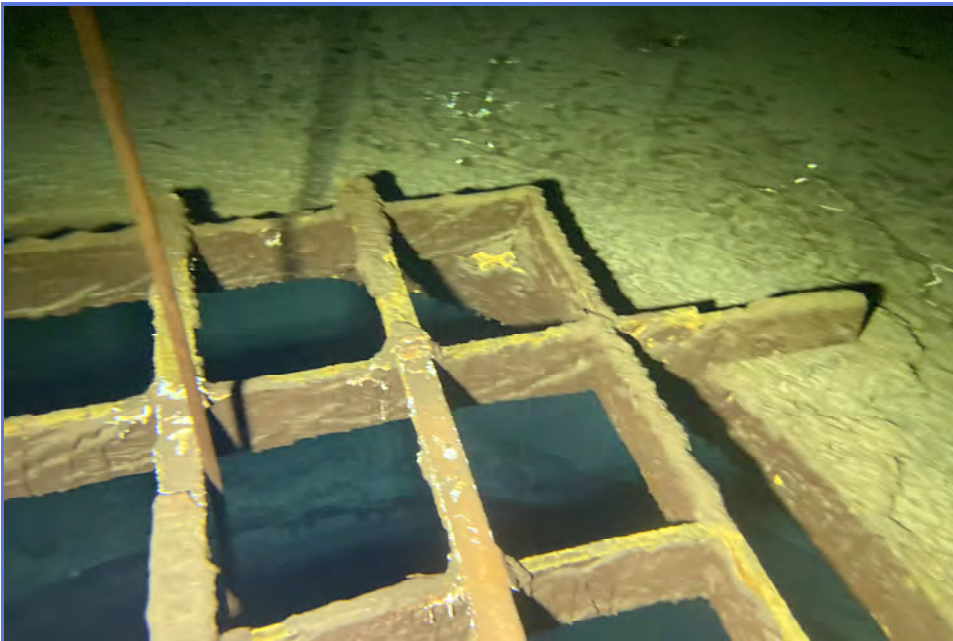
INTERIOR - City of Madera - 1MG Elevated Tank - Maintenance Inspection -070
