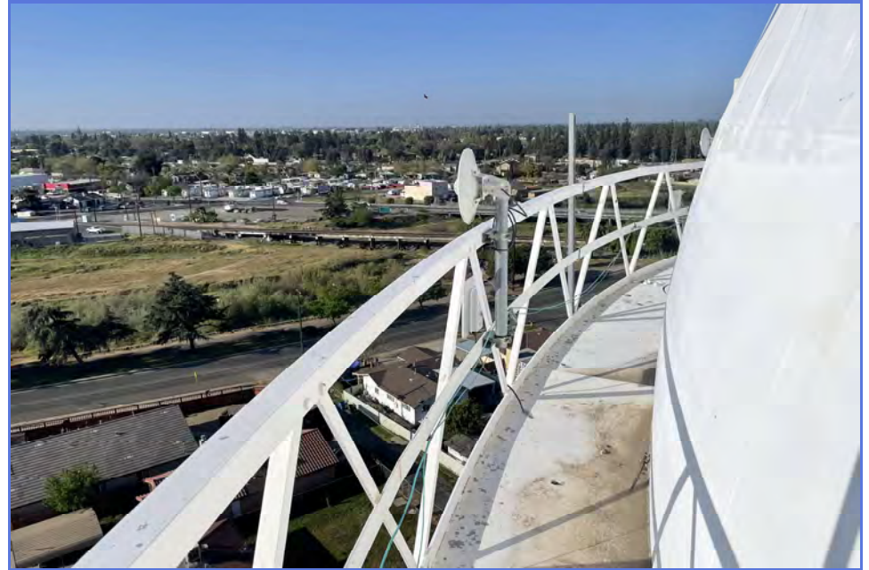
EXTERIOR - City of Madera - 1MG Elevated Tank - Maintenance Inspection -057
