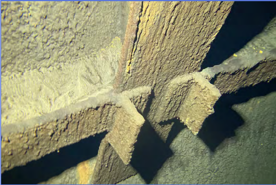
INTERIOR - City of Madera - 1MG Elevated Tank - Maintenance Inspection -040
