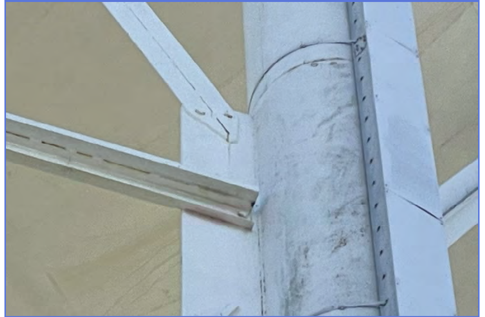
EXTERIOR - City of Madera - 1MG Elevated Tank - Maintenance Inspection -081
