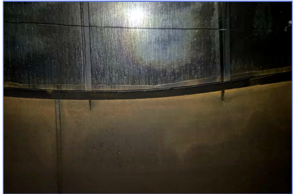
INTERIOR - City of Madera - 1MG Elevated Tank - Maintenance Inspection -007
