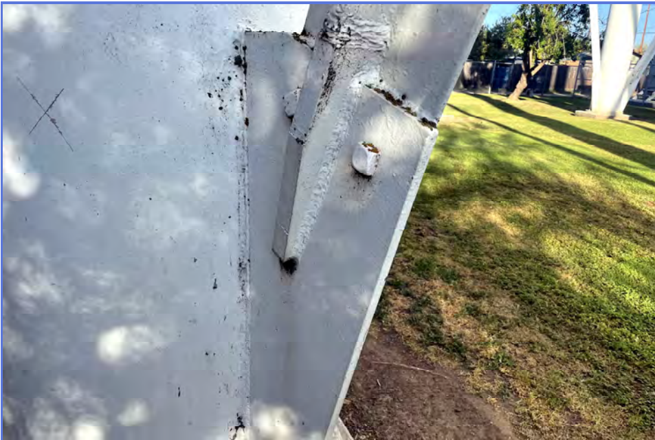
EXTERIOR - City of Madera - 1MG Elevated Tank - Maintenance Inspection -090
