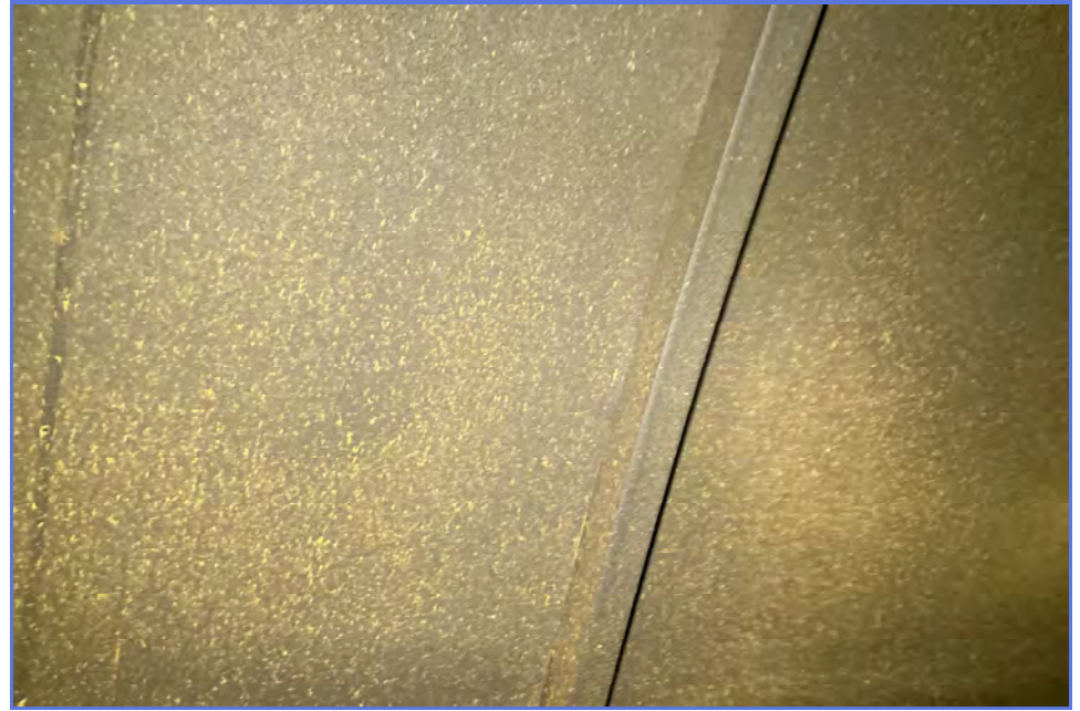
INTERIOR - City of Madera - 1MG Elevated Tank - Maintenance Inspection -025
