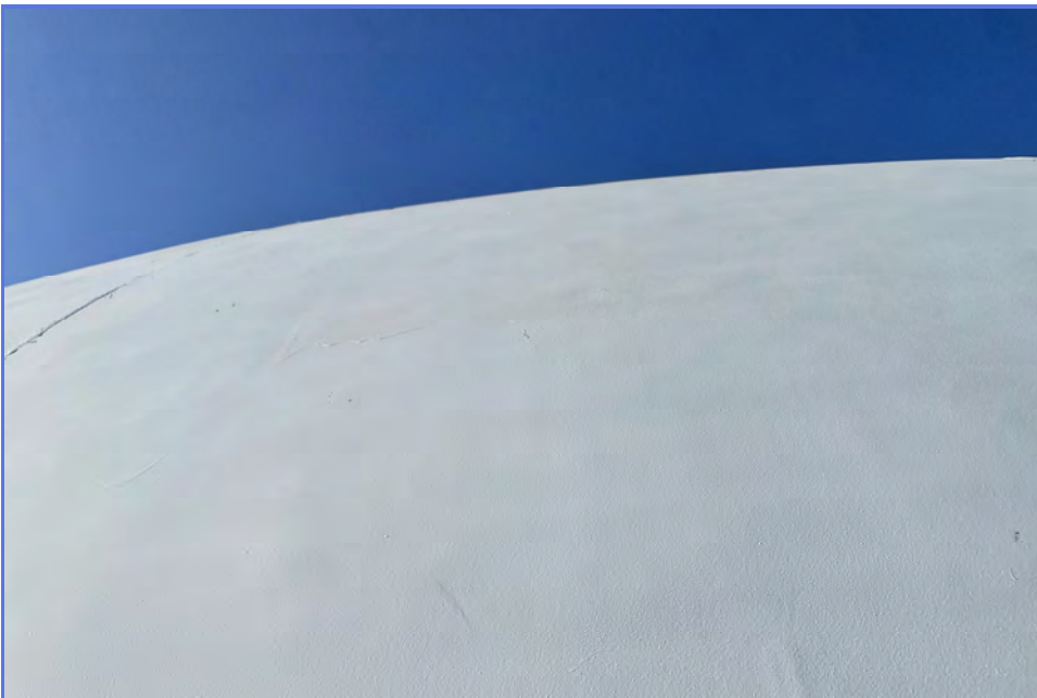
EXTERIOR - City of Madera - 1MG Elevated Tank - Maintenance Inspection -030
