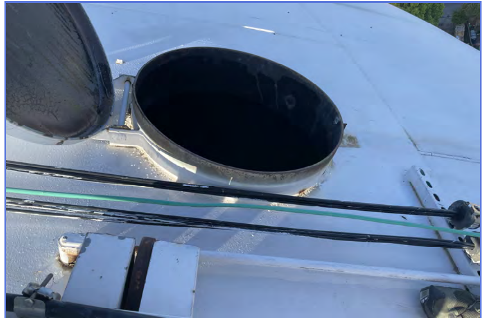
EXTERIOR - City of Madera - 1MG Elevated Tank - Maintenance Inspection -007
