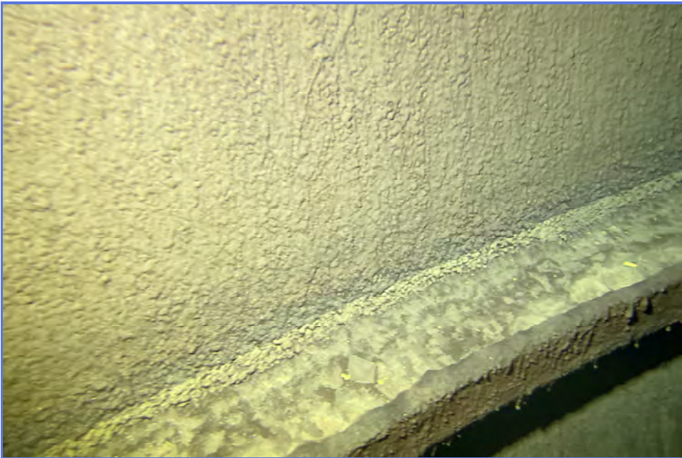
INTERIOR - City of Madera - 1MG Elevated Tank - Maintenance Inspection -030
