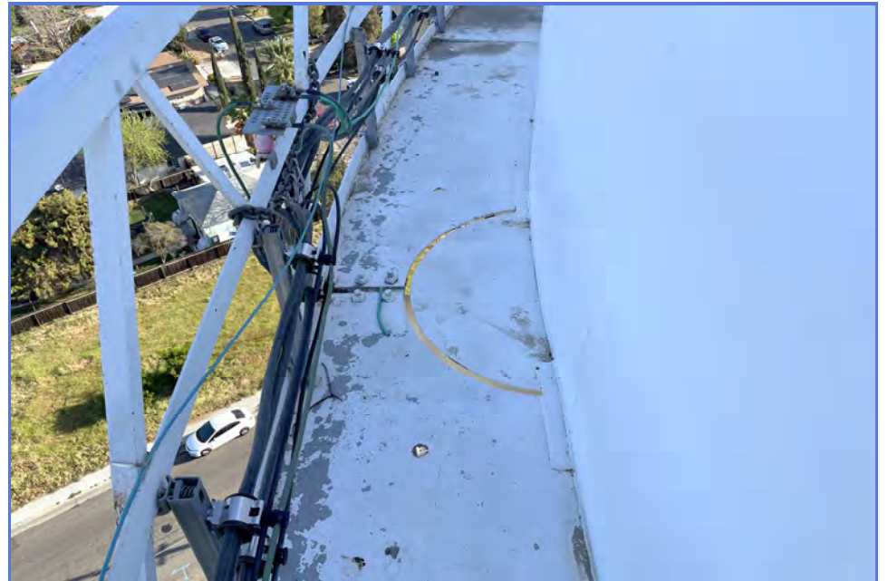
EXTERIOR - City of Madera - 1MG Elevated Tank - Maintenance Inspection -055
