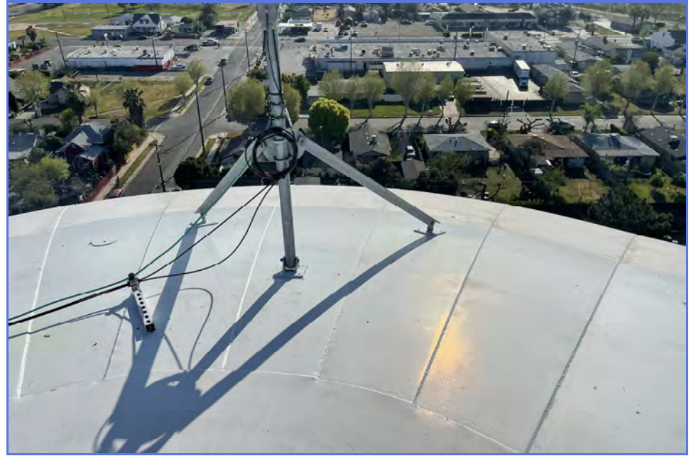
EXTERIOR - City of Madera - 1MG Elevated Tank - Maintenance Inspection -001
