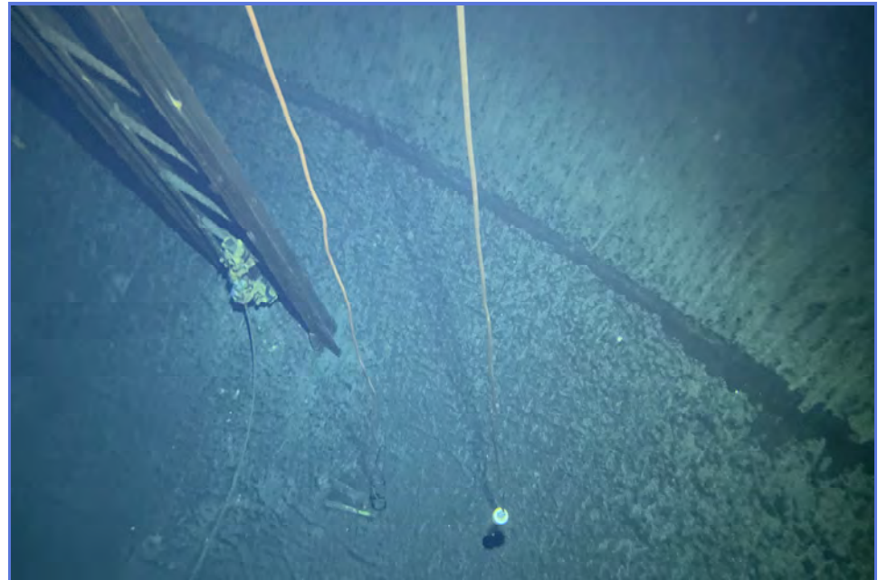
INTERIOR - City of Madera - 1MG Elevated Tank - Maintenance Inspection -075
