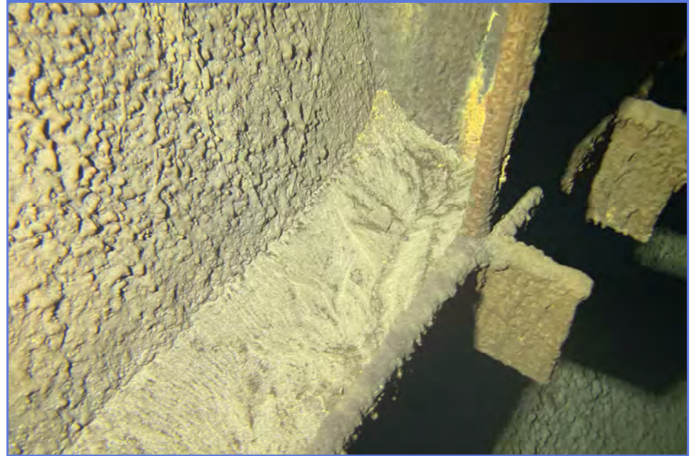
INTERIOR - City of Madera - 1MG Elevated Tank - Maintenance Inspection -041
