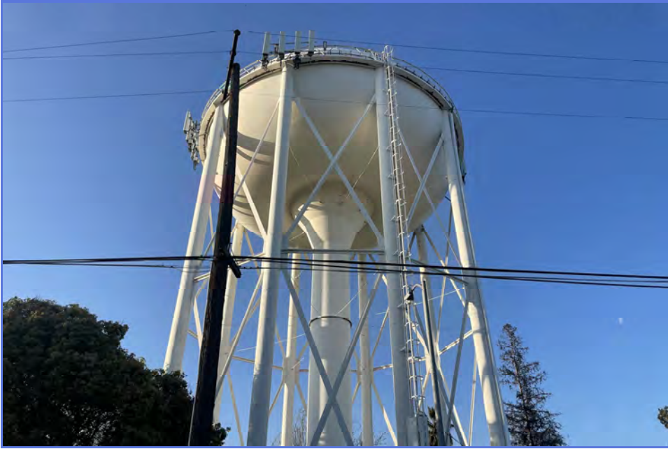
EXTERIOR - City of Madera - 1MG Elevated Tank - Maintenance Inspection -
