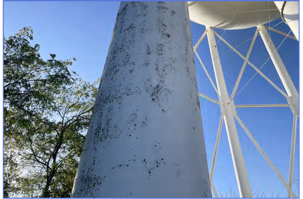
EXTERIOR - City of Madera - 1MG Elevated Tank - Maintenance Inspection -093
