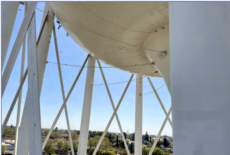
EXTERIOR - City of Madera - 1MG Elevated Tank - Maintenance Inspection -066
