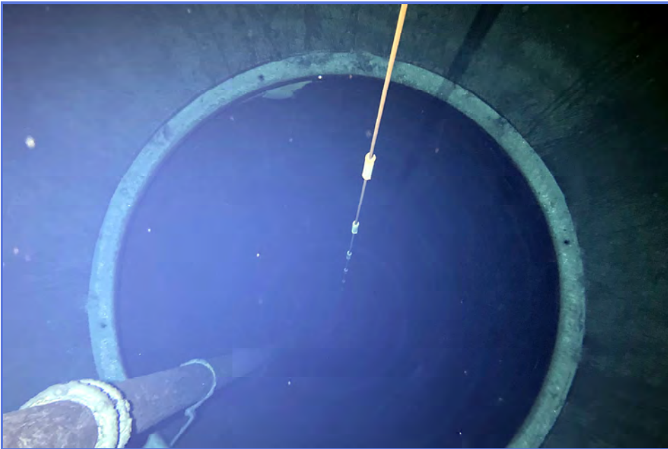
INTERIOR - City of Madera - 1MG Elevated Tank - Maintenance Inspection -062
