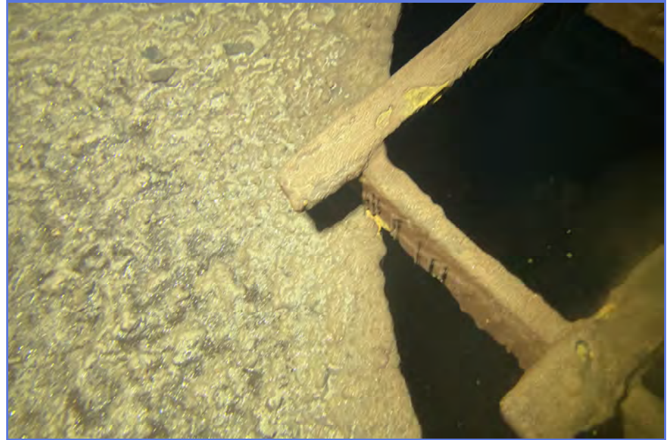
INTERIOR - City of Madera - 1MG Elevated Tank - Maintenance Inspection -069
