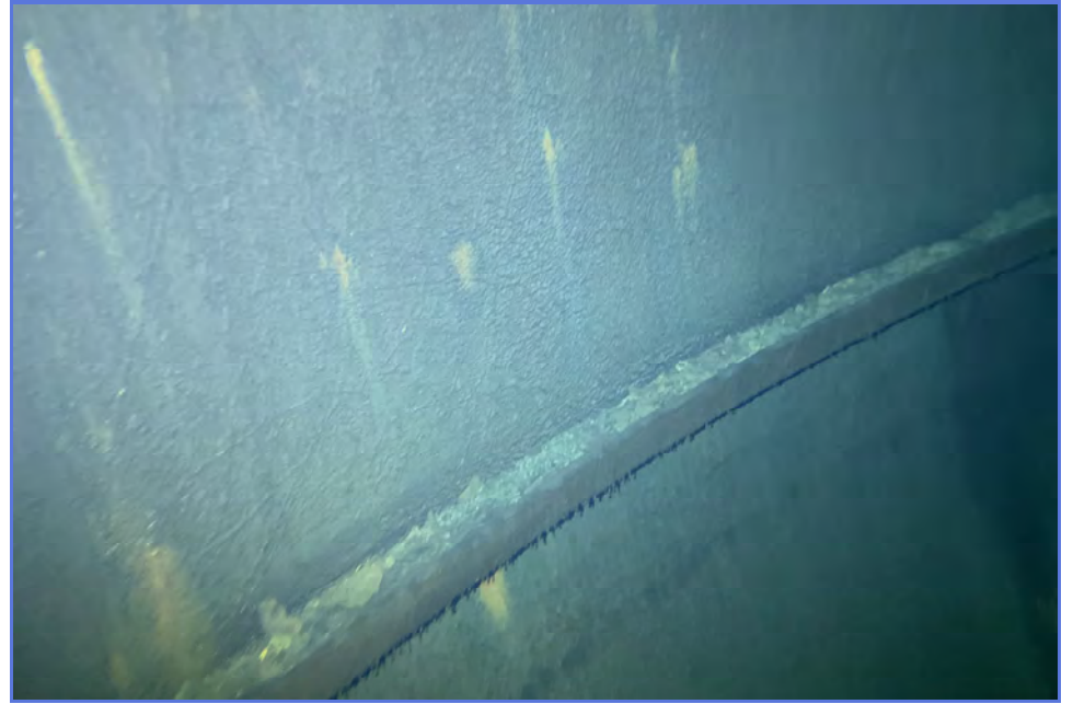
INTERIOR - City of Madera - 1MG Elevated Tank - Maintenance Inspection -045
