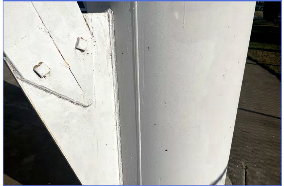
EXTERIOR - City of Madera - 1MG Elevated Tank - Maintenance Inspection -097
