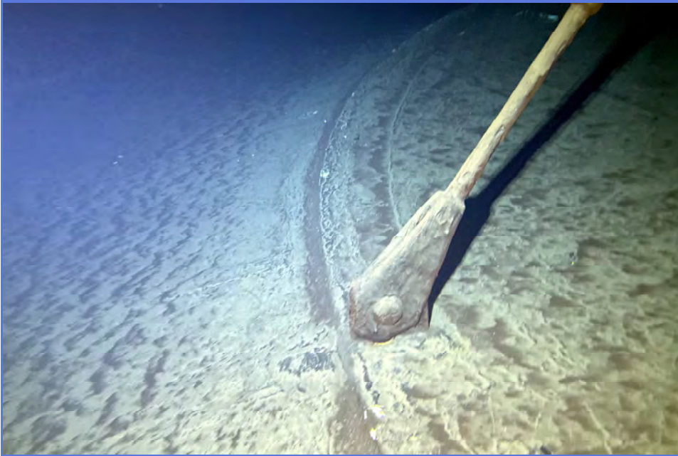
INTERIOR - City of Madera - 1MG Elevated Tank - Maintenance Inspection -064
