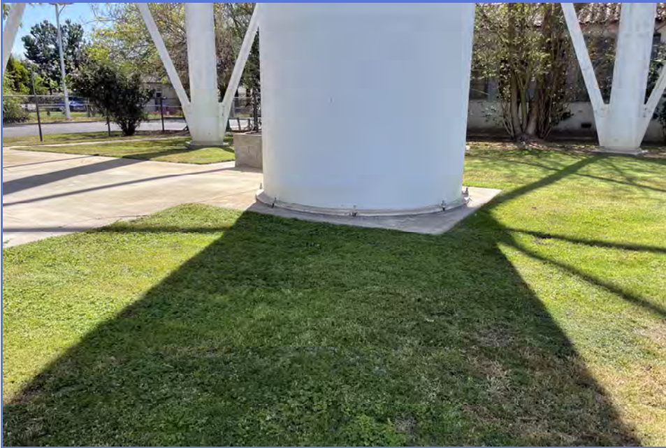
EXTERIOR - City of Madera - 1MG Elevated Tank - Maintenance Inspection -088
