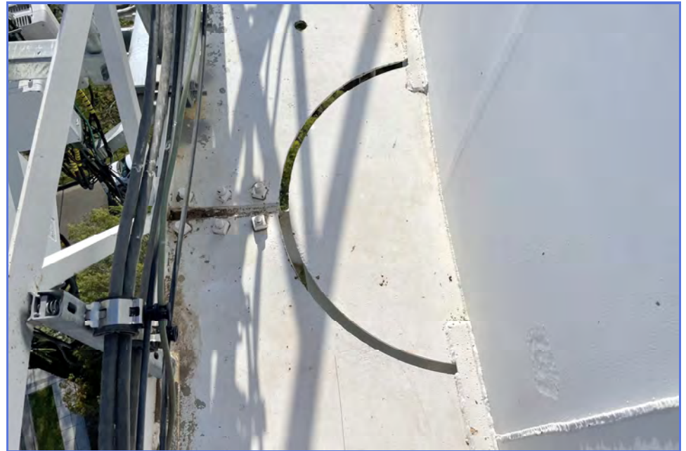
EXTERIOR - City of Madera - 1MG Elevated Tank - Maintenance Inspection -051
