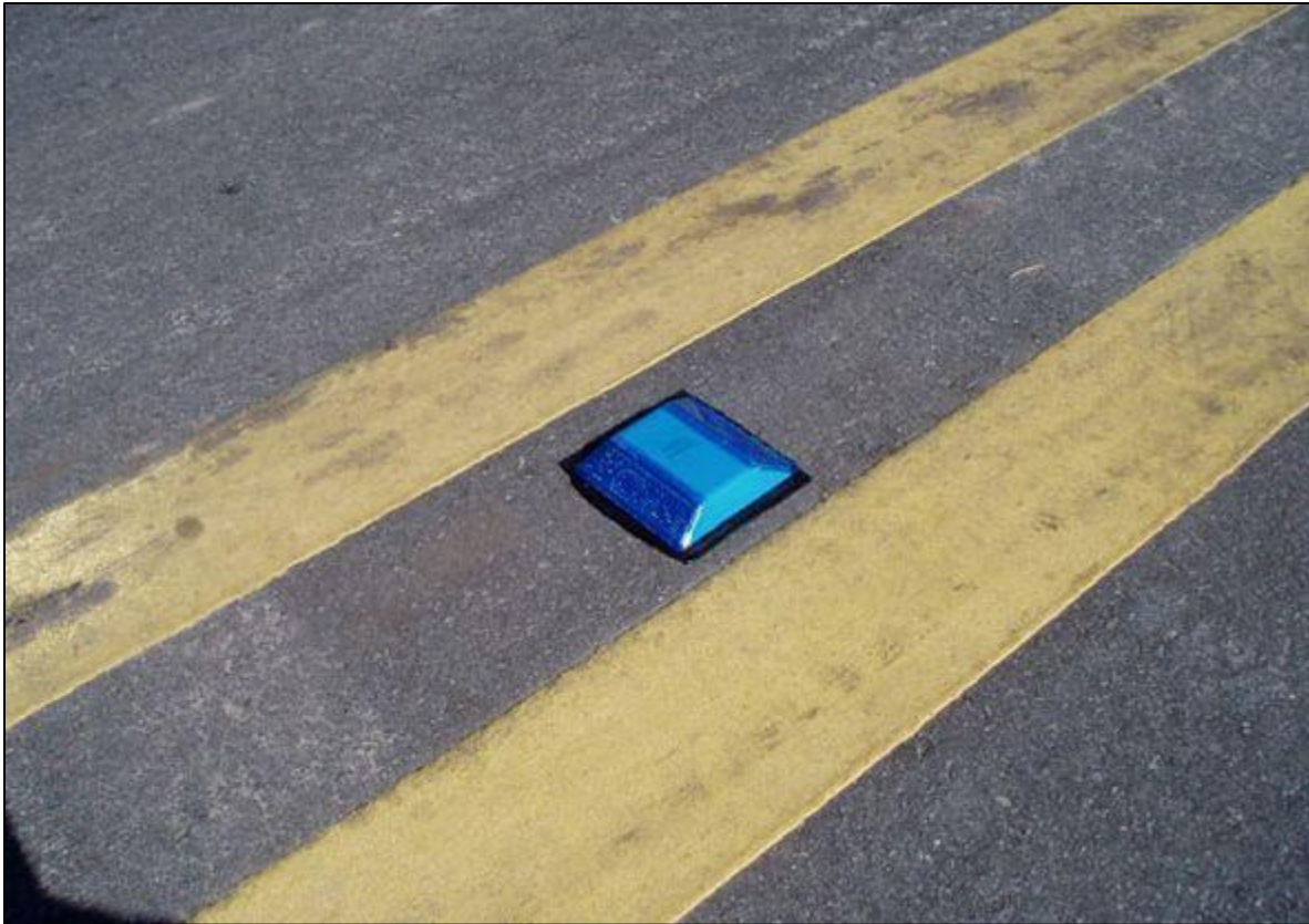
Attachment 1: Example of a blue street reflector signifying the location of a fire hydrant
