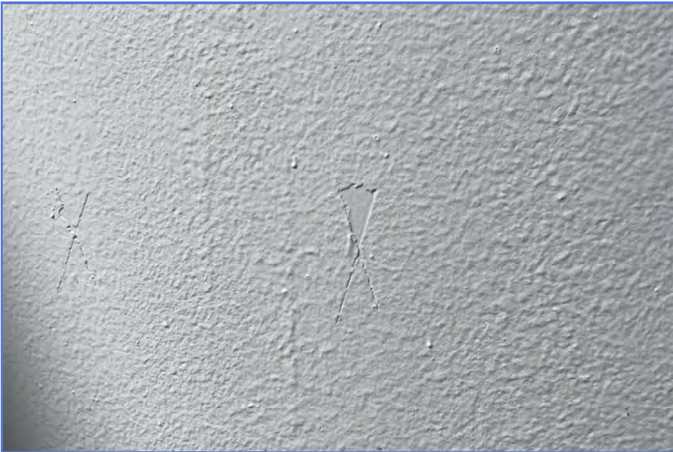
EXTERIOR - City of Madera - 1MG Elevated Tank - Maintenance Inspection -042
