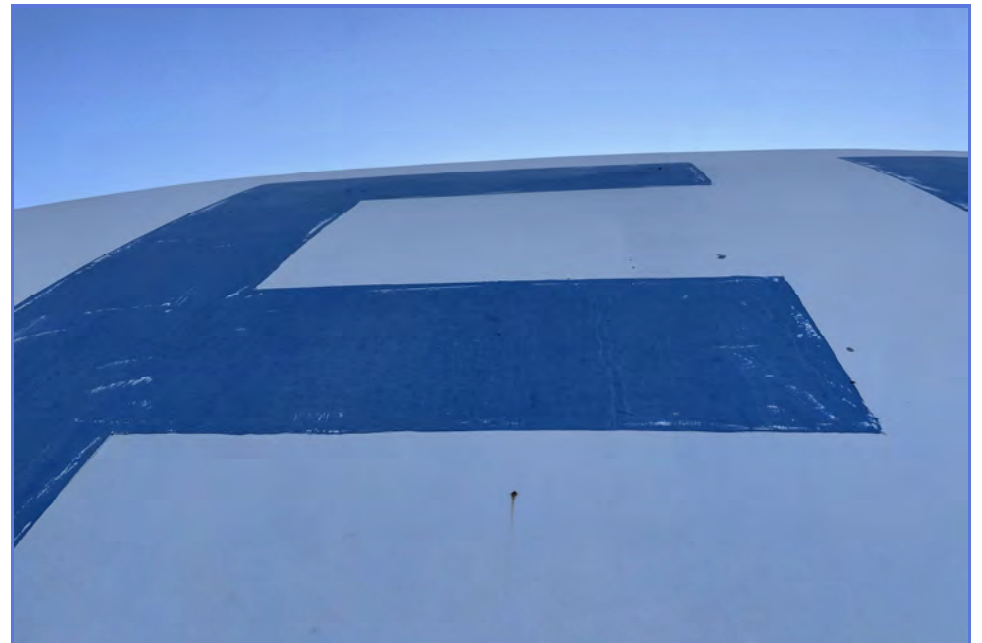
EXTERIOR - City of Madera - 1MG Elevated Tank - Maintenance Inspection -011
