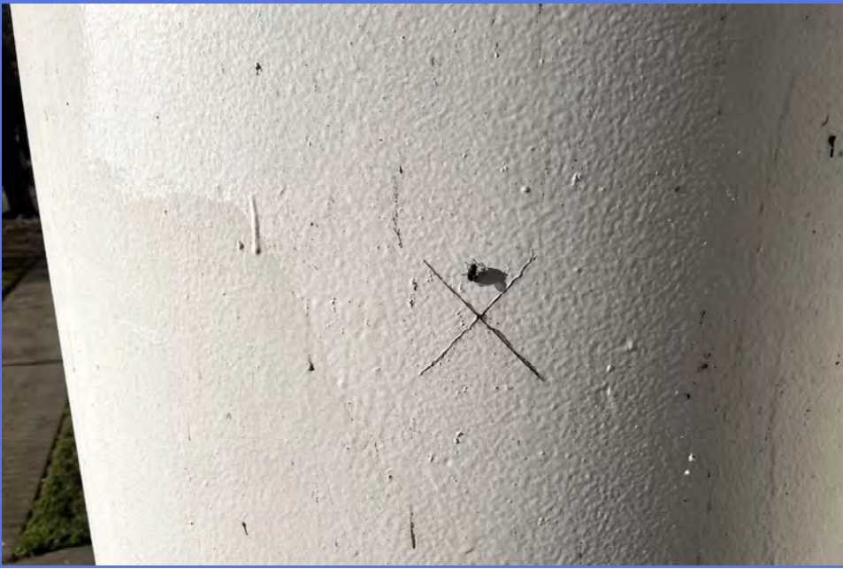
EXTERIOR - City of Madera - 1MG Elevated Tank - Maintenance Inspection -092
