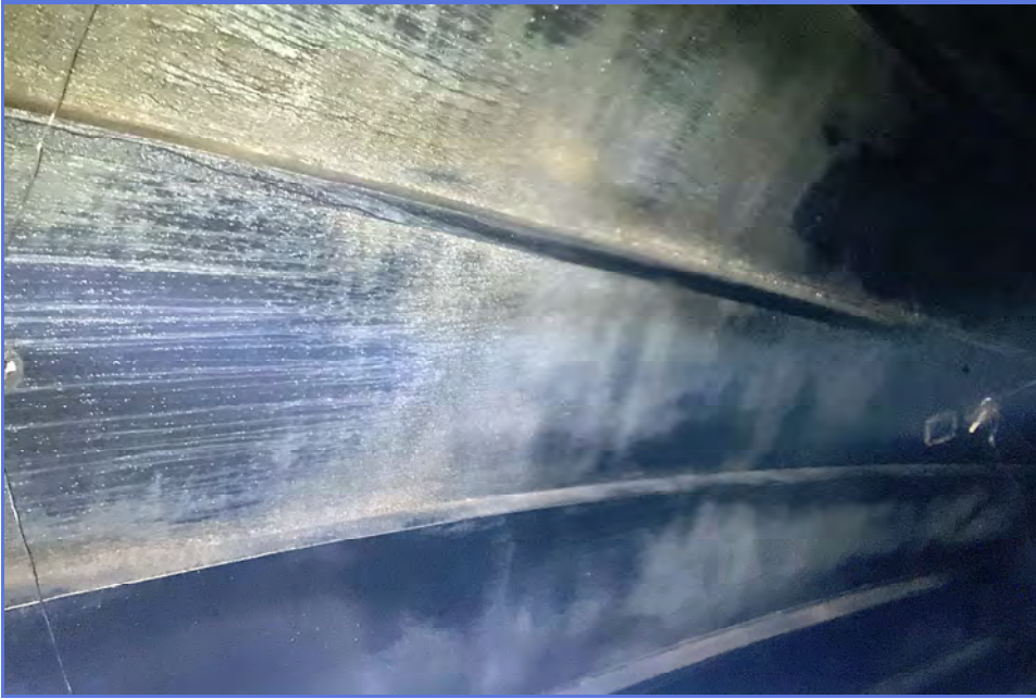
INTERIOR - City of Madera - 1MG Elevated Tank - Maintenance Inspection -004
