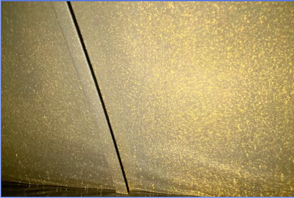
INTERIOR - City of Madera - 1MG Elevated Tank - Maintenance Inspection -024
