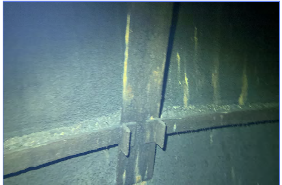
INTERIOR - City of Madera - 1MG Elevated Tank - Maintenance Inspection -039
