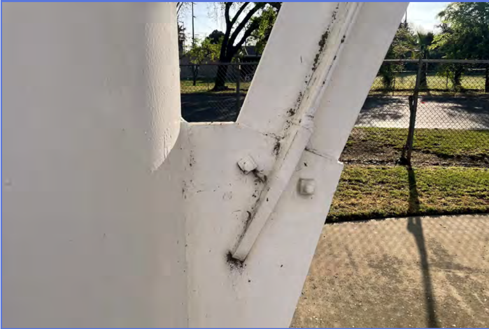
EXTERIOR - City of Madera - 1MG Elevated Tank - Maintenance Inspection -100
