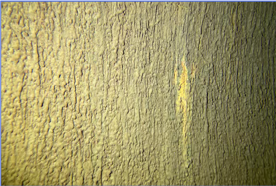
INTERIOR - City of Madera - 1MG Elevated Tank - Maintenance Inspection -054
