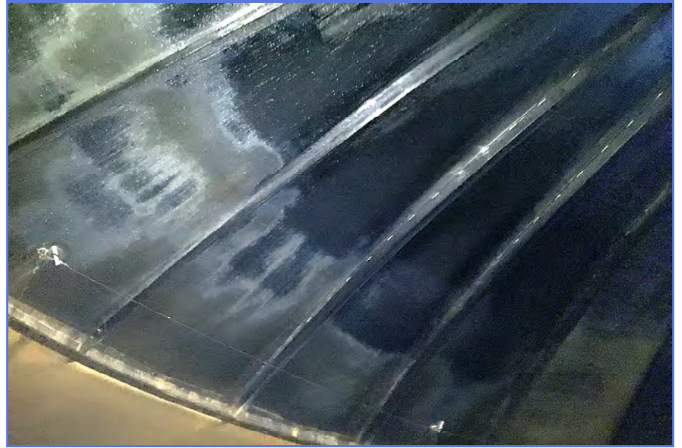
INTERIOR - City of Madera - 1MG Elevated Tank - Maintenance Inspection -005
