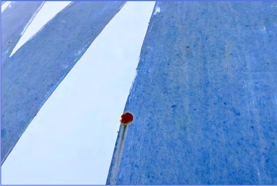
EXTERIOR - City of Madera - 1MG Elevated Tank - Maintenance Inspection -024
