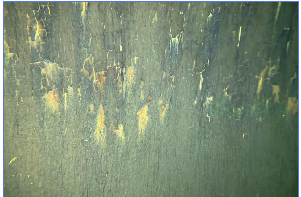
INTERIOR - City of Madera - 1MG Elevated Tank - Maintenance Inspection -051
