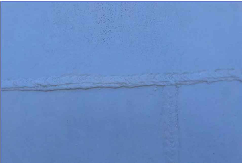
EXTERIOR - City of Madera - 1MG Elevated Tank - Maintenance Inspection -046
