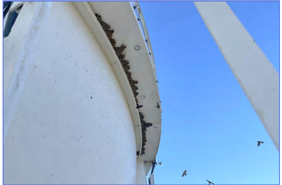
EXTERIOR - City of Madera - 1MG Elevated Tank - Maintenance Inspection -069
