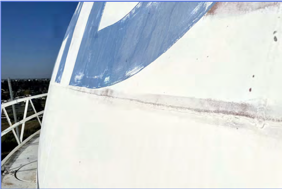
EXTERIOR - City of Madera - 1MG Elevated Tank - Maintenance Inspection -022
