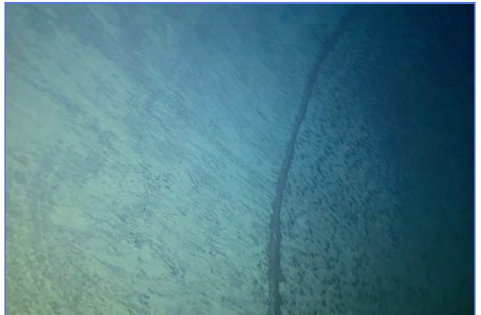
INTERIOR - City of Madera - 1MG Elevated Tank - Maintenance Inspection -059
