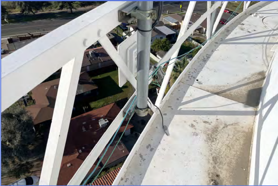
EXTERIOR - City of Madera - 1MG Elevated Tank - Maintenance Inspection -056
