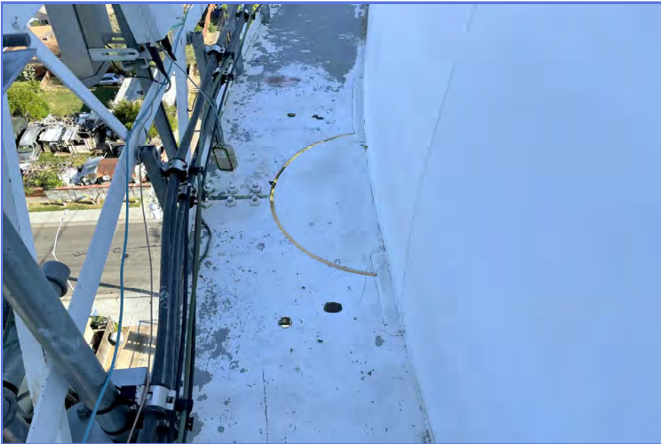
EXTERIOR - City of Madera - 1MG Elevated Tank - Maintenance Inspection -050
