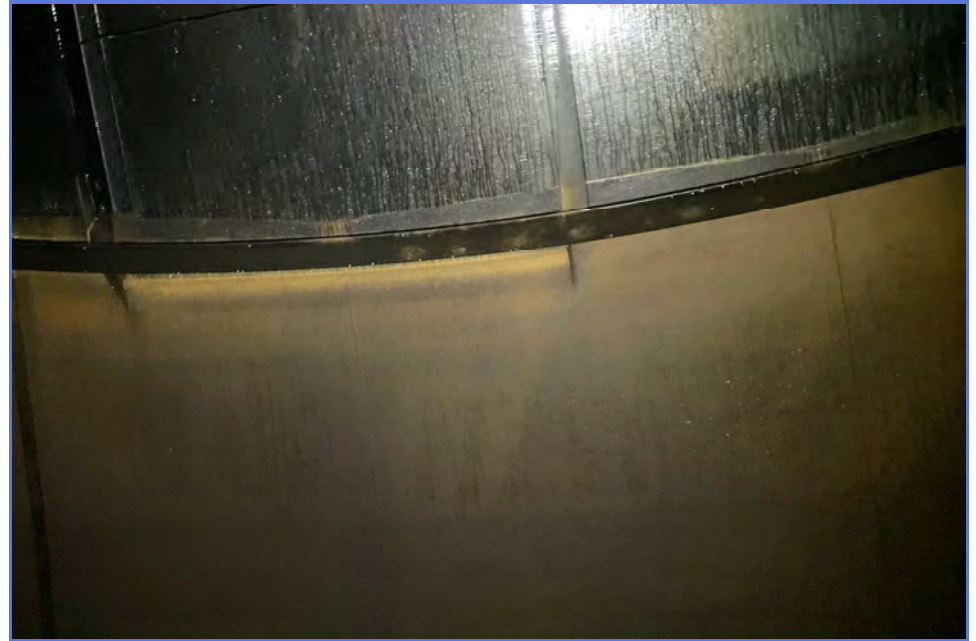
INTERIOR - City of Madera - 1MG Elevated Tank - Maintenance Inspection -013
