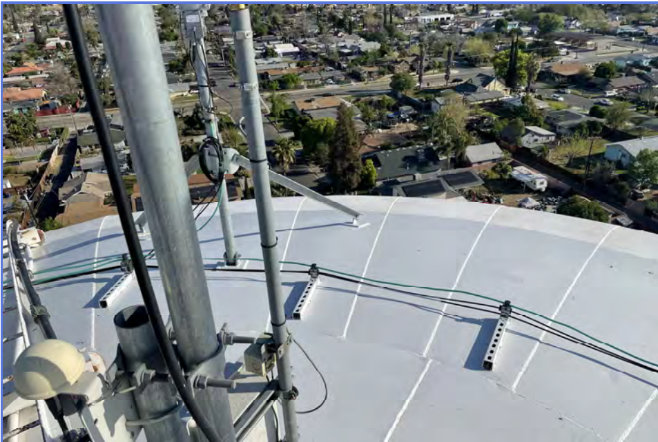
EXTERIOR - City of Madera - 1MG Elevated Tank - Maintenance Inspection -006
