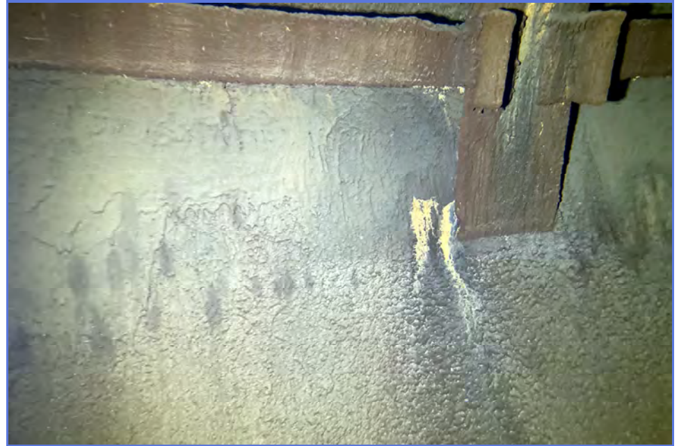
INTERIOR - City of Madera - 1MG Elevated Tank - Maintenance Inspection -037
