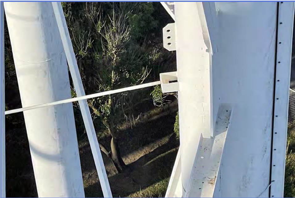
EXTERIOR - City of Madera - 1MG Elevated Tank - Maintenance Inspection -074
