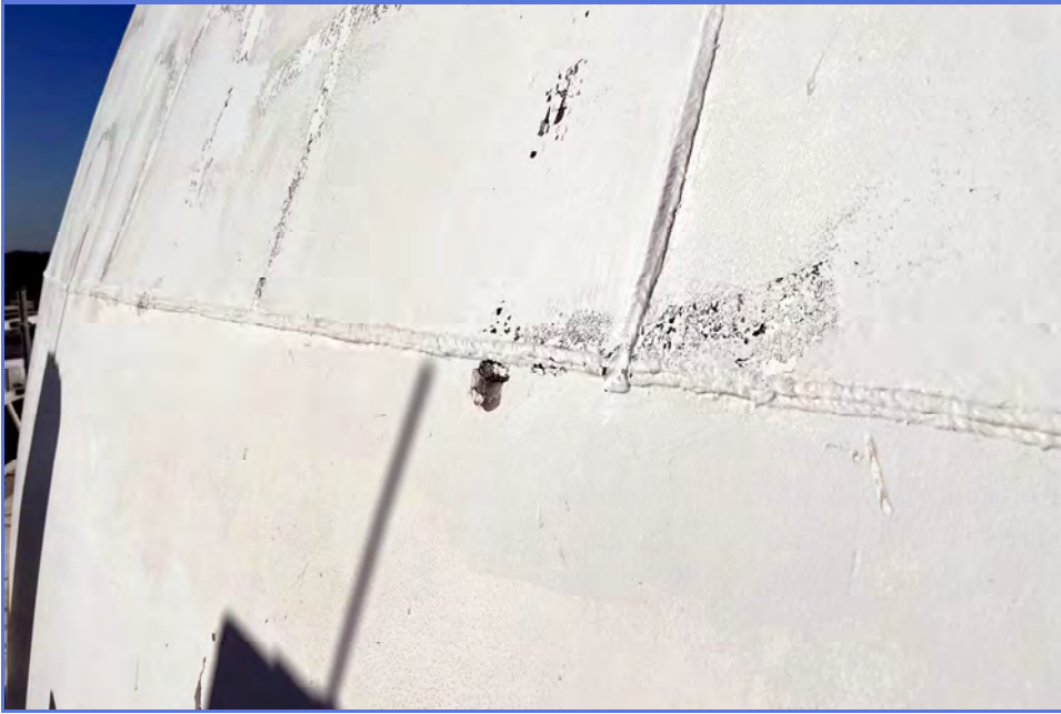
EXTERIOR - City of Madera - 1MG Elevated Tank - Maintenance Inspection -040
