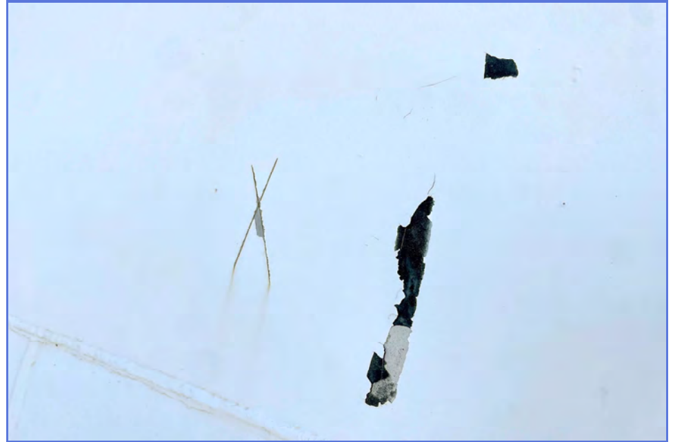
EXTERIOR - City of Madera - 1MG Elevated Tank - Maintenance Inspection -049
