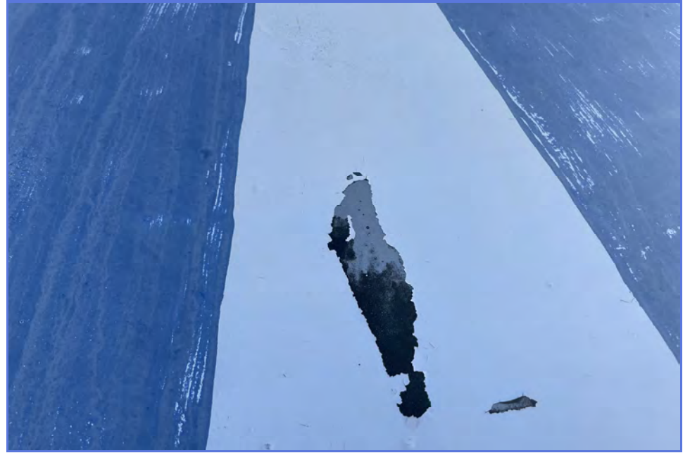
EXTERIOR - City of Madera - 1MG Elevated Tank - Maintenance Inspection -017
