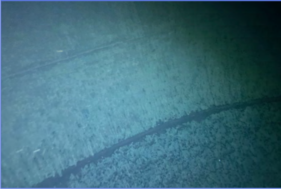
INTERIOR - City of Madera - 1MG Elevated Tank - Maintenance Inspection -060
