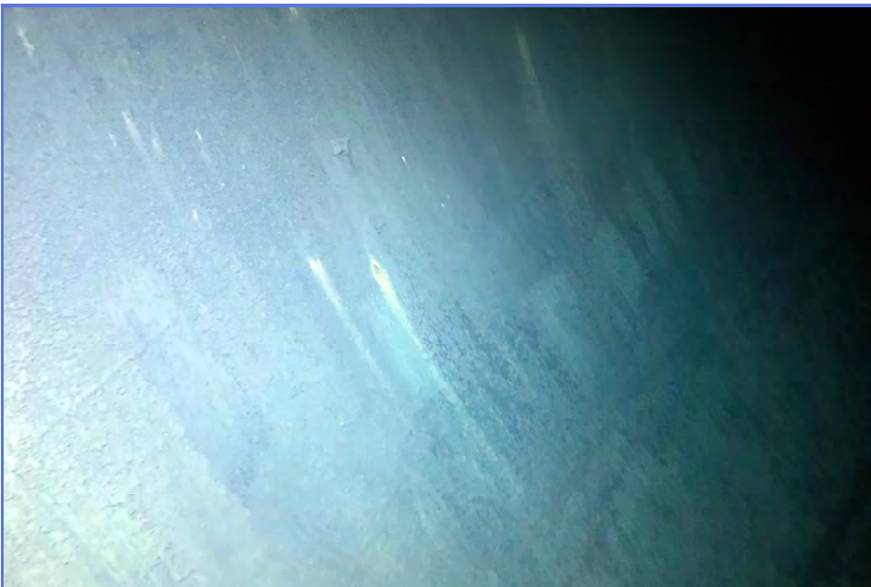
INTERIOR - City of Madera - 1MG Elevated Tank - Maintenance Inspection -058
