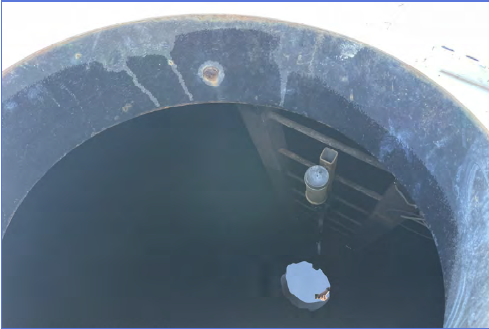
EXTERIOR - City of Madera - 1MG Elevated Tank - Maintenance Inspection -008
