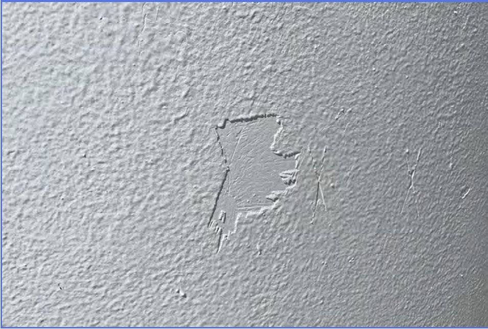
EXTERIOR - City of Madera - 1MG Elevated Tank - Maintenance Inspection -044
