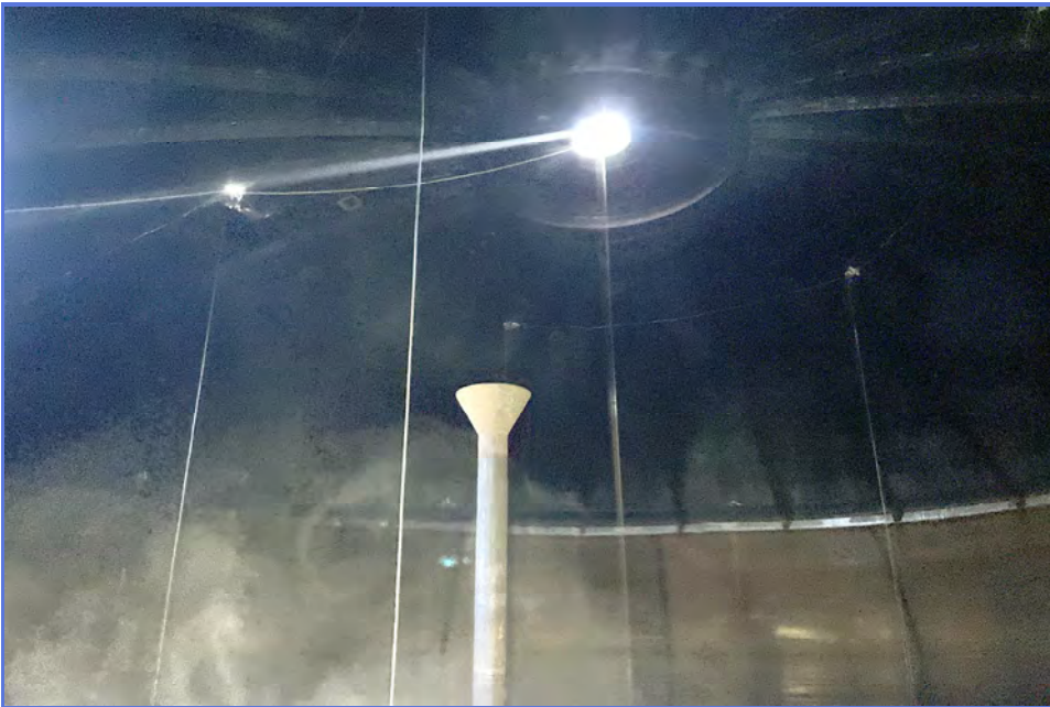
INTERIOR - City of Madera - 1MG Elevated Tank - Maintenance Inspection -002
