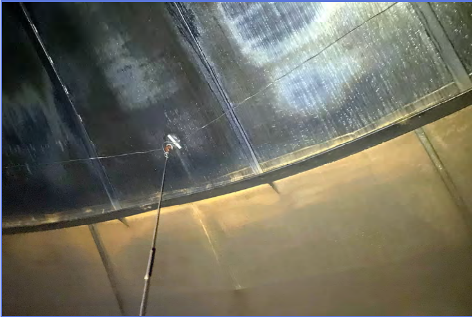
INTERIOR - City of Madera - 1MG Elevated Tank - Maintenance Inspection -008
