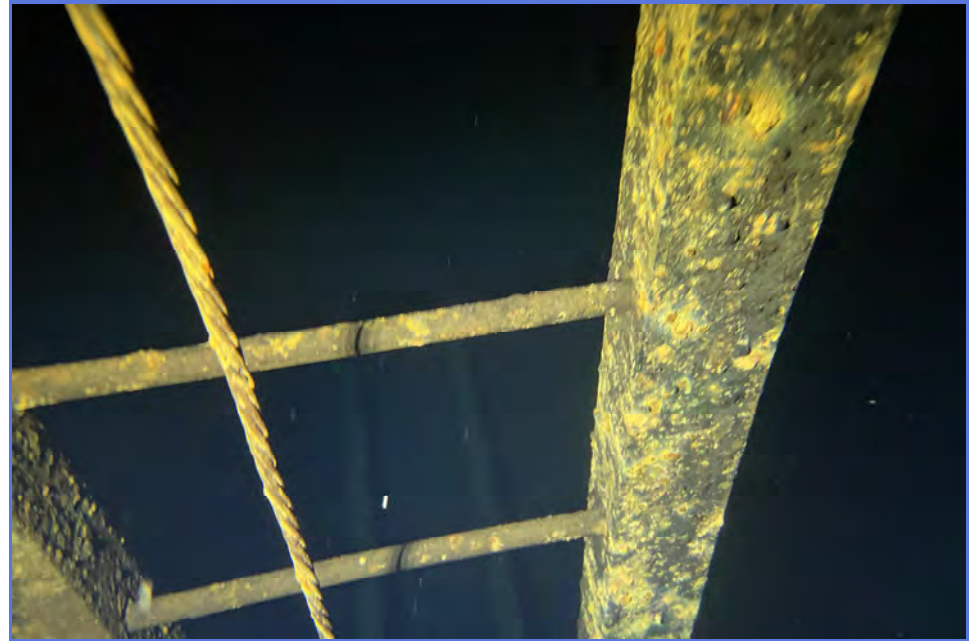
INTERIOR - City of Madera - 1MG Elevated Tank - Maintenance Inspection -073
