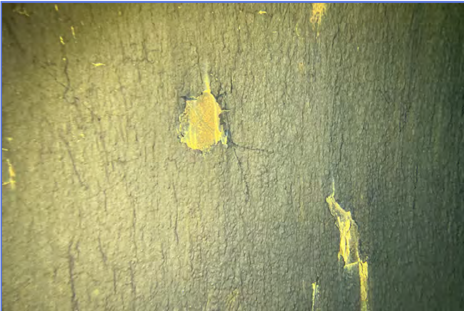
INTERIOR - City of Madera - 1MG Elevated Tank - Maintenance Inspection -050
