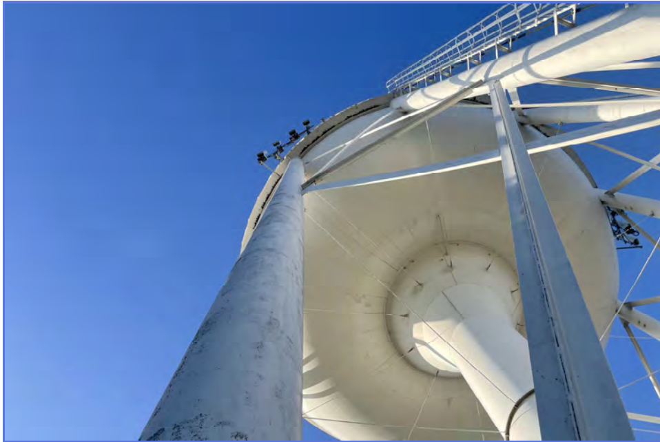
EXTERIOR - City of Madera - 1MG Elevated Tank - Maintenance Inspection -084
