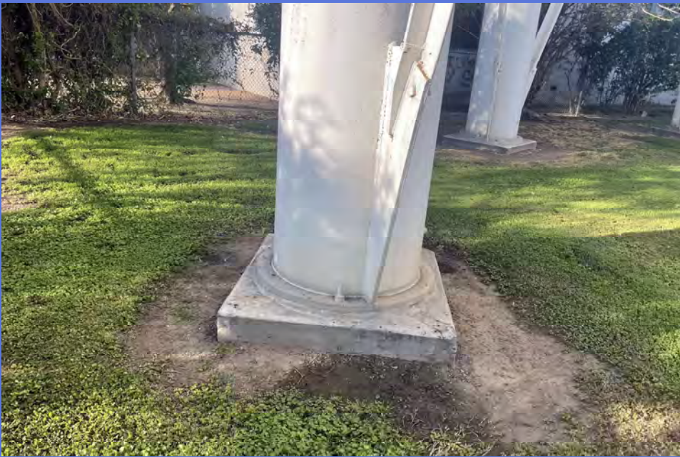
EXTERIOR - City of Madera - 1MG Elevated Tank - Maintenance Inspection -094
