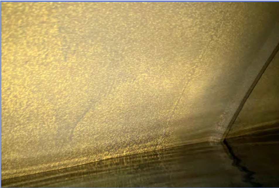
INTERIOR - City of Madera - 1MG Elevated Tank - Maintenance Inspection -022
