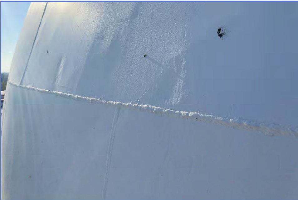
EXTERIOR - City of Madera - 1MG Elevated Tank - Maintenance Inspection -034
