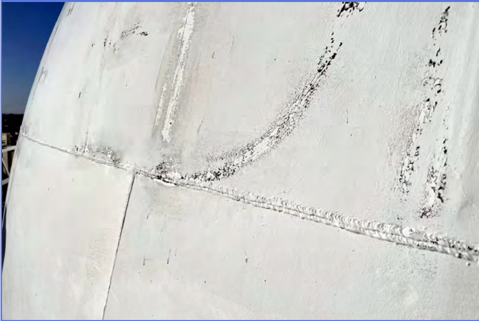
EXTERIOR - City of Madera - 1MG Elevated Tank - Maintenance Inspection -048
