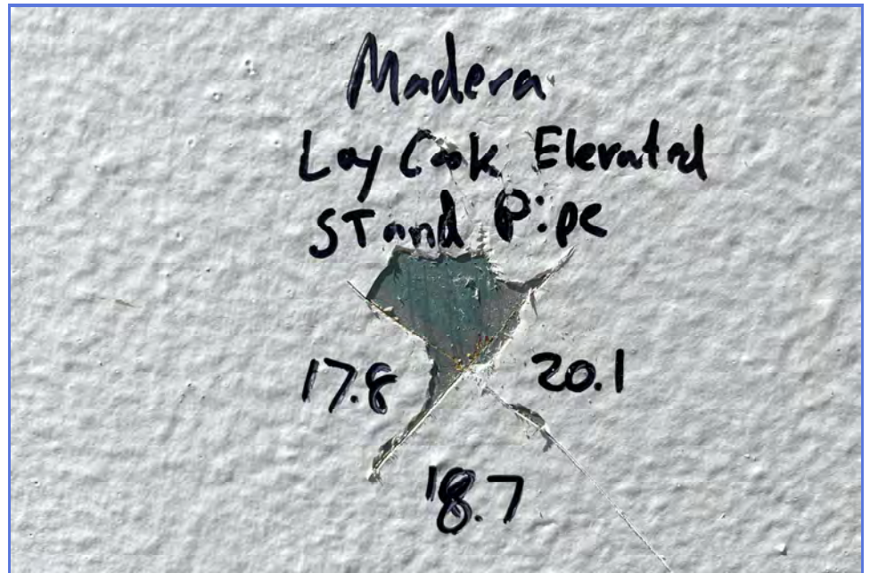
EXTERIOR - City of Madera - 1MG Elevated Tank - Maintenance Inspection -087
