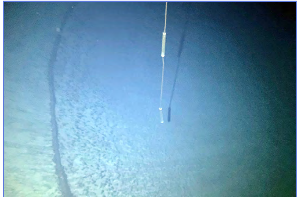
INTERIOR - City of Madera - 1MG Elevated Tank - Maintenance Inspection -063
