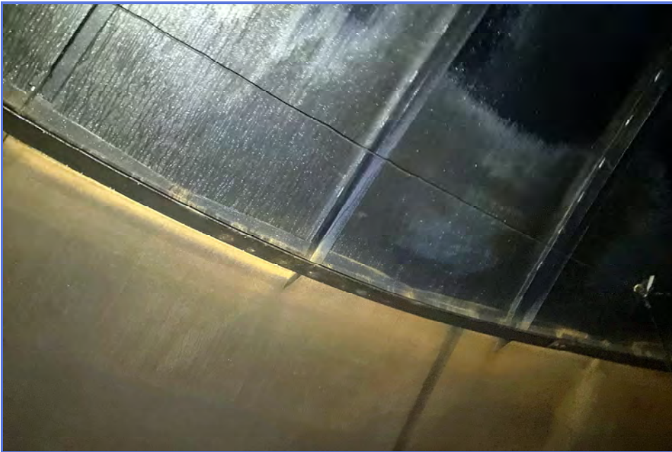
INTERIOR - City of Madera - 1MG Elevated Tank - Maintenance Inspection -006
