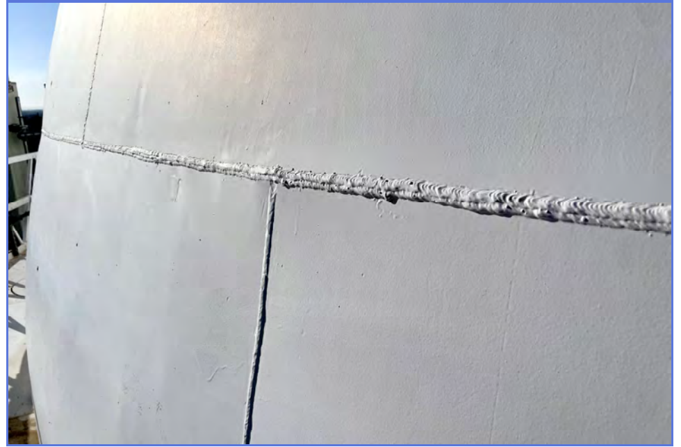
EXTERIOR - City of Madera - 1MG Elevated Tank - Maintenance Inspection -037
