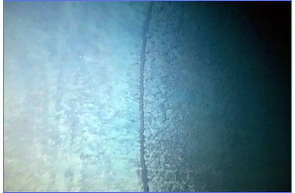
INTERIOR - City of Madera - 1MG Elevated Tank - Maintenance Inspection -061
