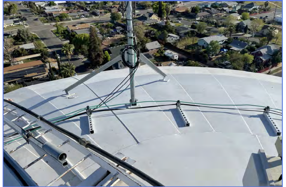
EXTERIOR - City of Madera - 1MG Elevated Tank - Maintenance Inspection -005
