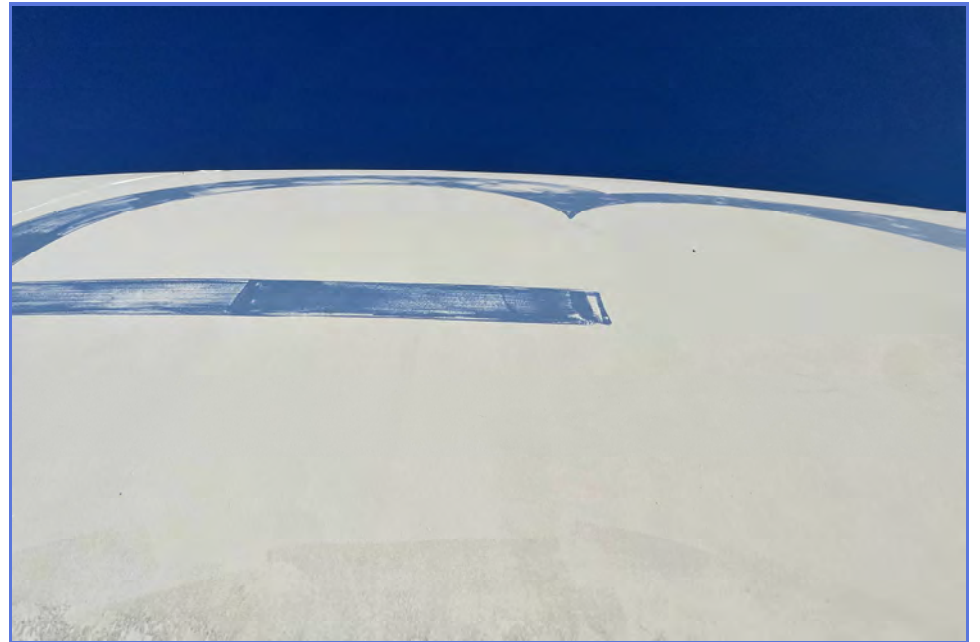
EXTERIOR - City of Madera - 1MG Elevated Tank - Maintenance Inspection -023
