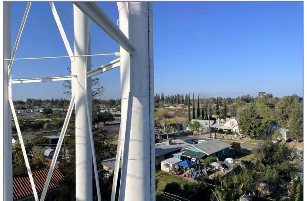
EXTERIOR - City of Madera - 1MG Elevated Tank - Maintenance Inspection -075
