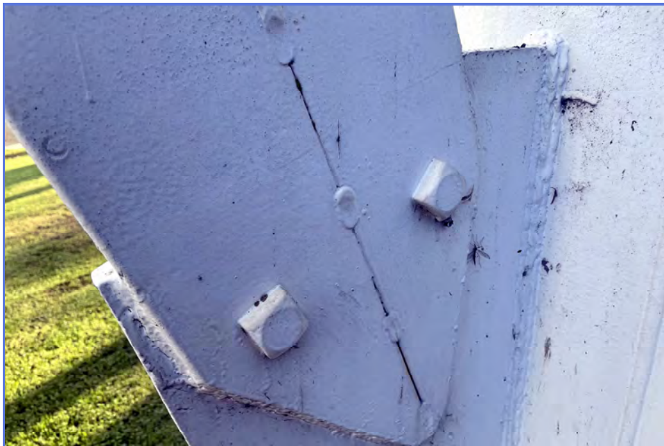
EXTERIOR - City of Madera - 1MG Elevated Tank - Maintenance Inspection -098
