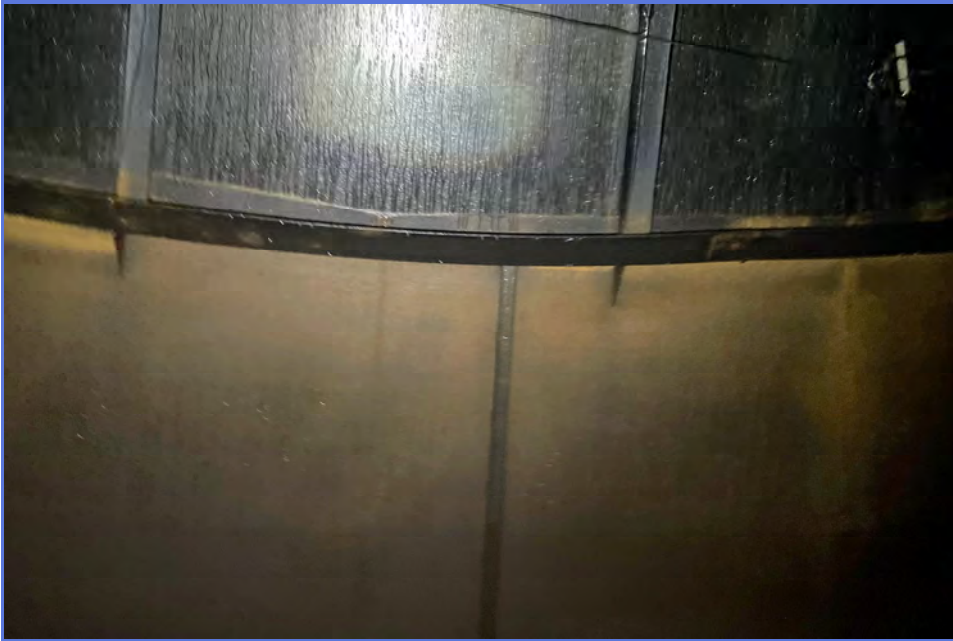
INTERIOR - City of Madera - 1MG Elevated Tank - Maintenance Inspection -012
