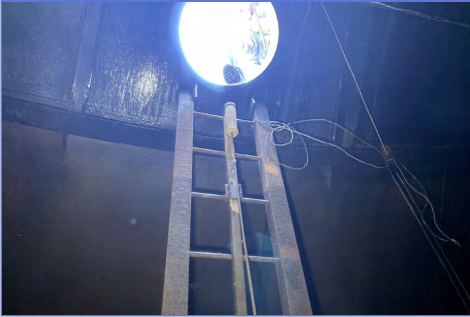
INTERIOR - City of Madera - 1MG Elevated Tank - Maintenance Inspection -
