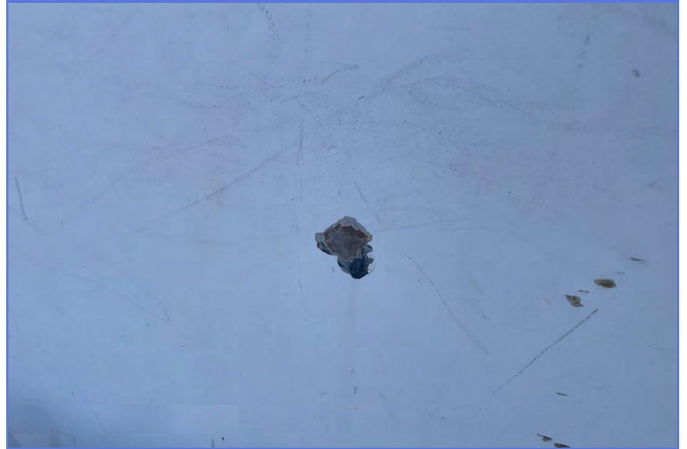
EXTERIOR - City of Madera - 1MG Elevated Tank - Maintenance Inspection -029
