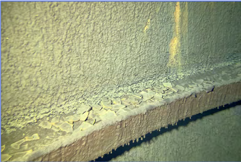
INTERIOR - City of Madera - 1MG Elevated Tank - Maintenance Inspection -046
