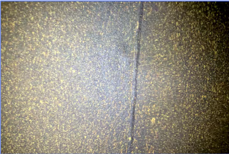
INTERIOR - City of Madera - 1MG Elevated Tank - Maintenance Inspection -018
