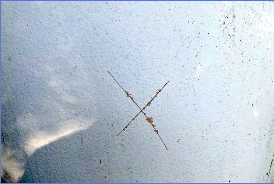
EXTERIOR - City of Madera - 1MG Elevated Tank - Maintenance Inspection -036
