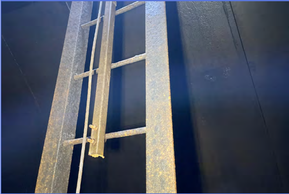
INTERIOR - City of Madera - 1MG Elevated Tank - Maintenance Inspection -072
