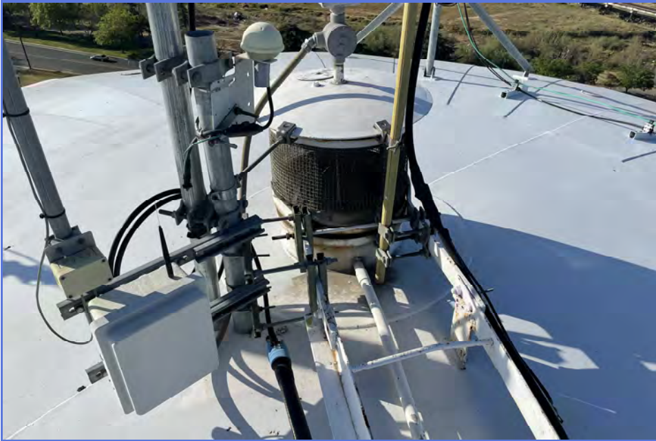
EXTERIOR - City of Madera - 1MG Elevated Tank - Maintenance Inspection -004
