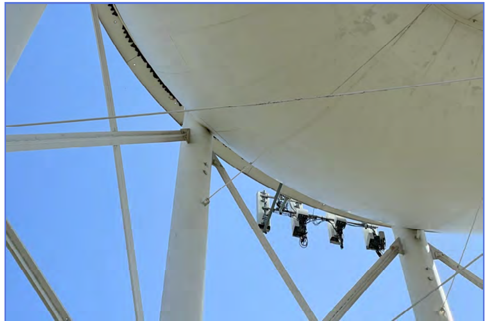
EXTERIOR - City of Madera - 1MG Elevated Tank - Maintenance Inspection -067
