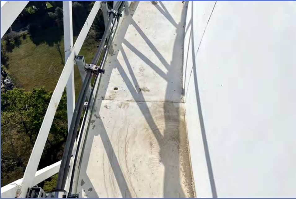
EXTERIOR - City of Madera - 1MG Elevated Tank - Maintenance Inspection -060
