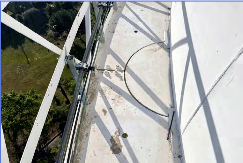
EXTERIOR - City of Madera - 1MG Elevated Tank - Maintenance Inspection -062
