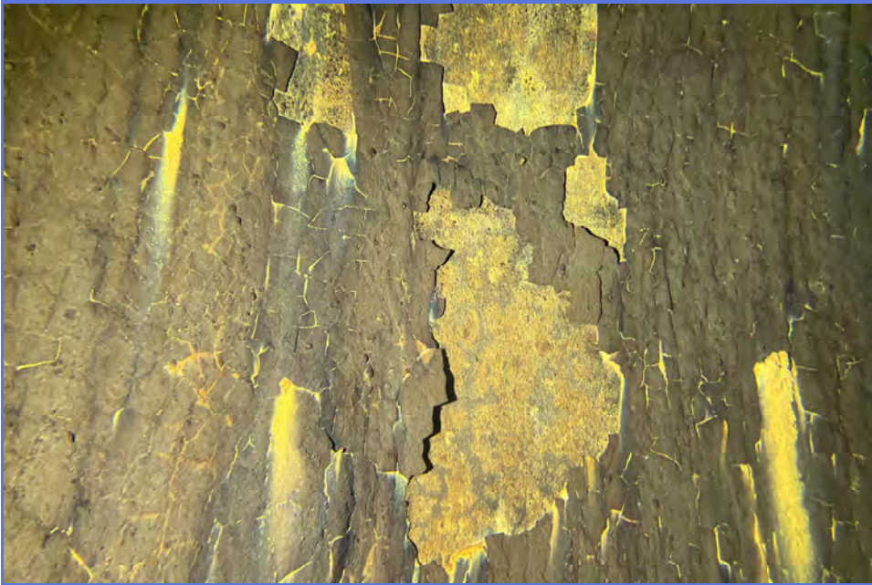
INTERIOR - City of Madera - 1MG Elevated Tank - Maintenance Inspection -048
