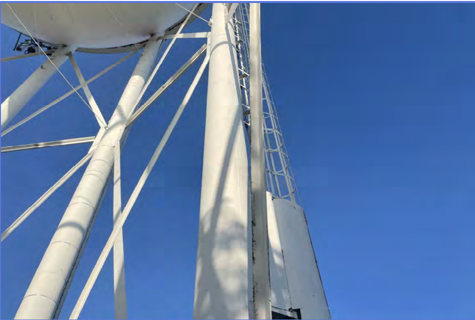
EXTERIOR - City of Madera - 1MG Elevated Tank - Maintenance Inspection -082
