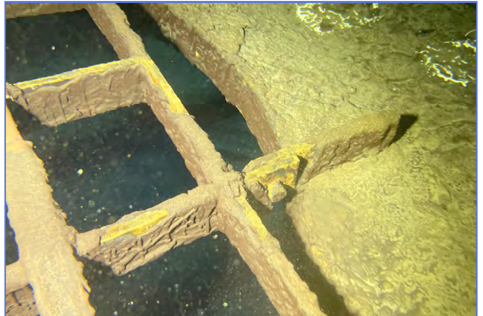
INTERIOR - City of Madera - 1MG Elevated Tank - Maintenance Inspection -067
