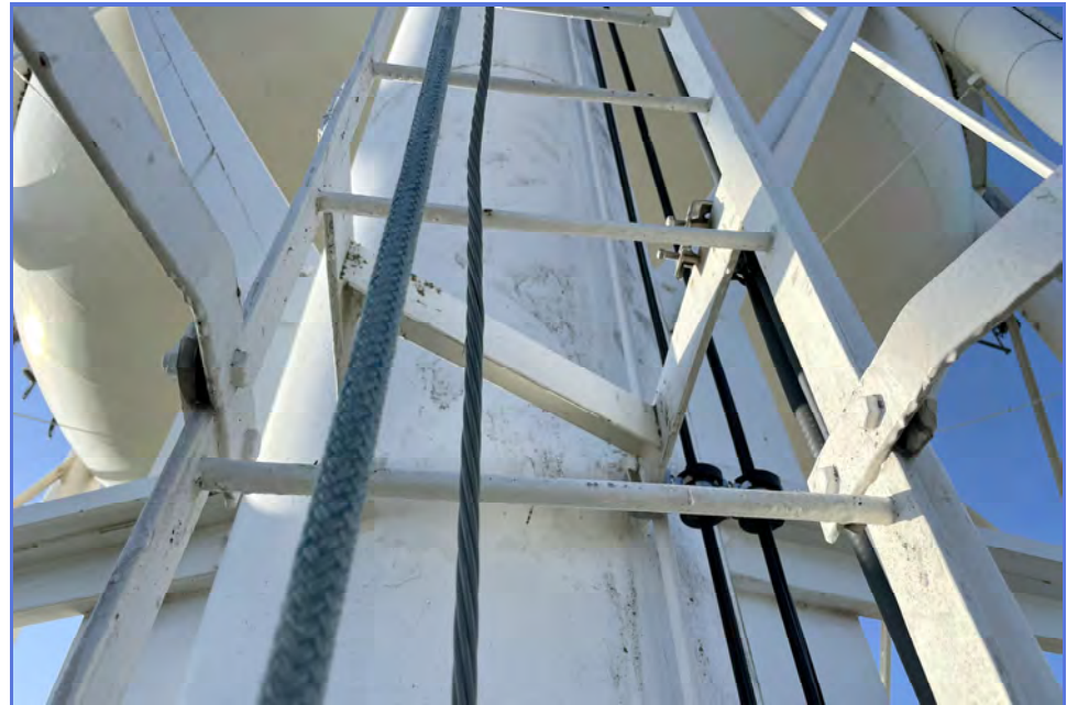
EXTERIOR - City of Madera - 1MG Elevated Tank - Maintenance Inspection -103
