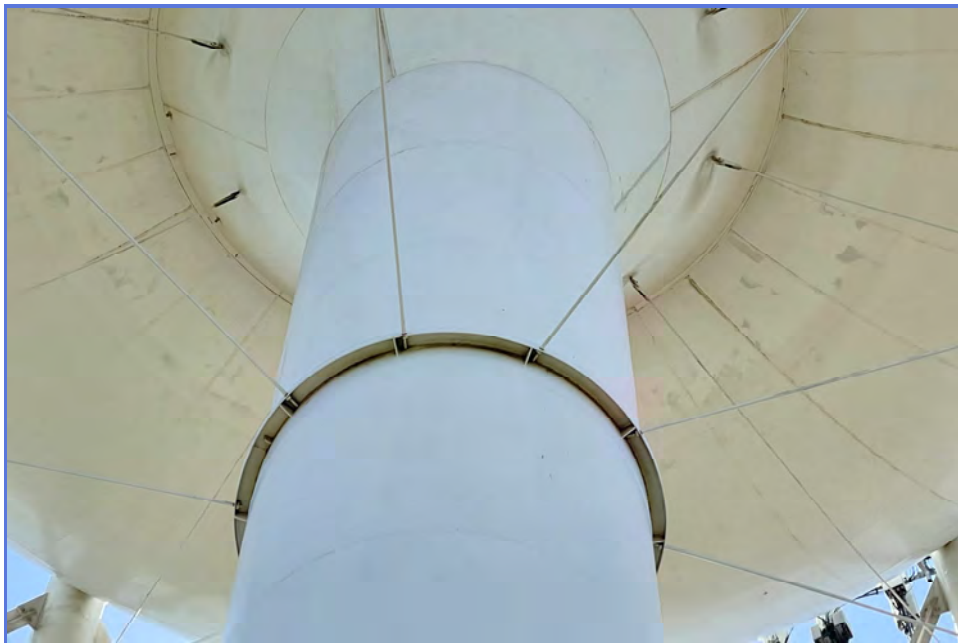
EXTERIOR - City of Madera - 1MG Elevated Tank - Maintenance Inspection -070
