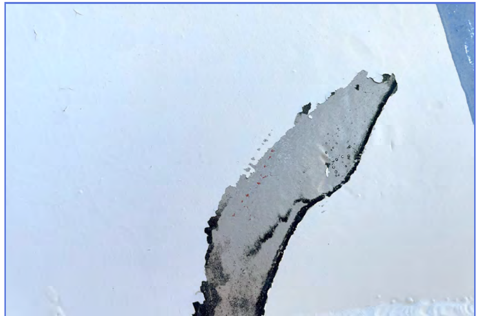
EXTERIOR - City of Madera - 1MG Elevated Tank - Maintenance Inspection -039
