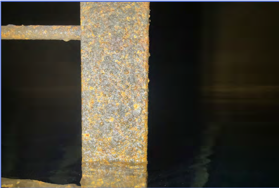
INTERIOR - City of Madera - 1MG Elevated Tank - Maintenance Inspection -026
