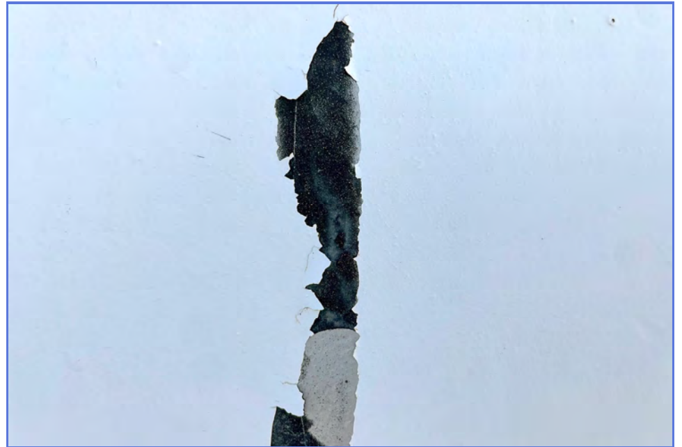
EXTERIOR - City of Madera - 1MG Elevated Tank - Maintenance Inspection -035
