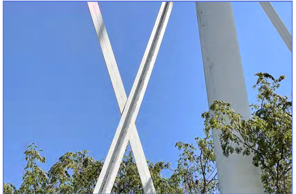
EXTERIOR - City of Madera - 1MG Elevated Tank - Maintenance Inspection -079
