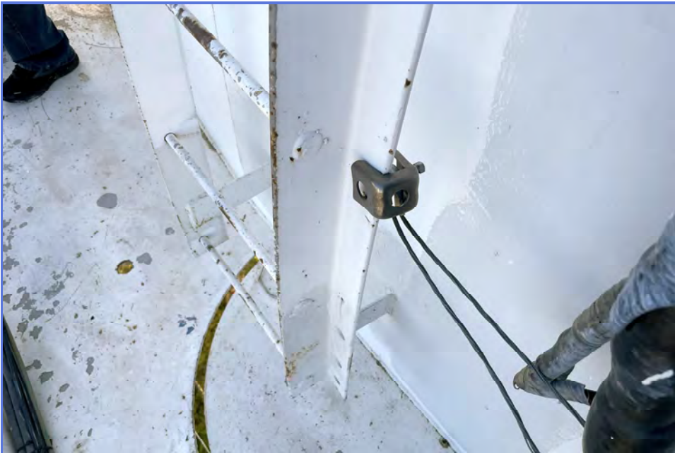
EXTERIOR - City of Madera - 1MG Elevated Tank - Maintenance Inspection -054
