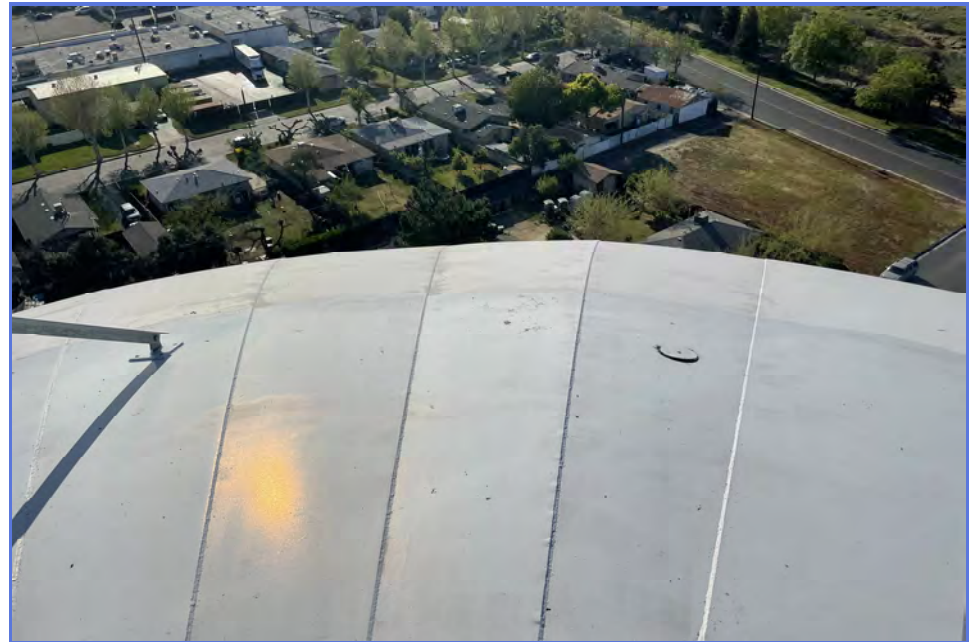
EXTERIOR - City of Madera - 1MG Elevated Tank - Maintenance Inspection -003
