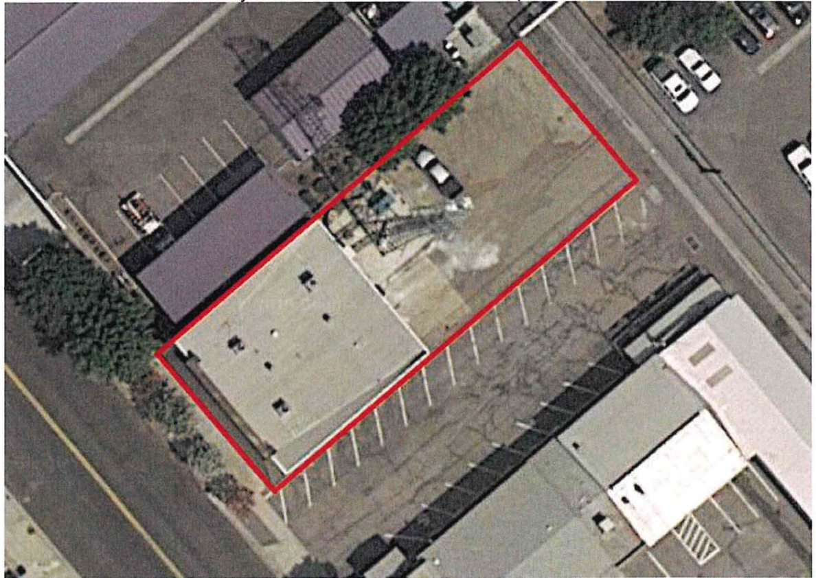
City of Madera – Madera Radio Dispatch site
