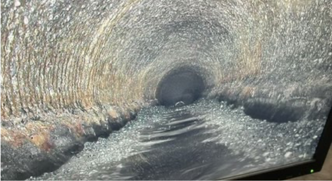
Figure 1 – Example of inside of pipe approximately 1/3 rd full of debris prior to cleaning
