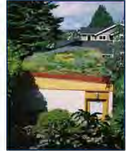
A "green roof" uses plant cover to provide insulation and reduce the heat generated by a standard roof.
