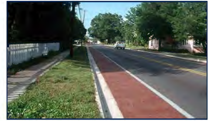
A "complete street" accommodates pedestrians (on the sidewalk), bicyclists (in an onstreet designated lane) and motorists.
