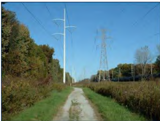
This utility corridor includes a walking trail.
