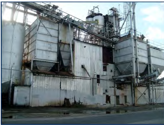
This facility near the downtown epitomizes the utilitarian character of many of Madera's industrial areas.
