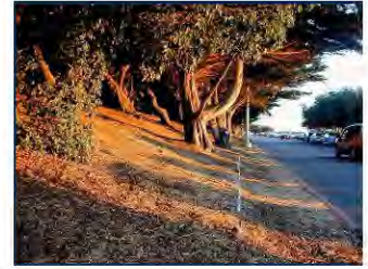
In this photo, a berm (left) is used in place of a wall to block roadway noise.
