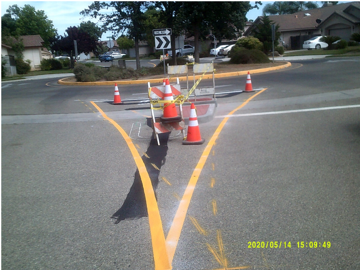
Figure 2 – South Raised Median
