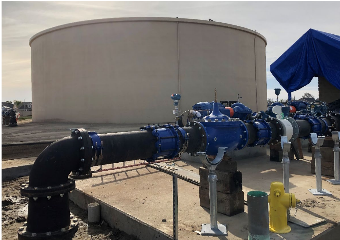
Figure 2 Concrete Tank and Booster Pump Station Under Construction
