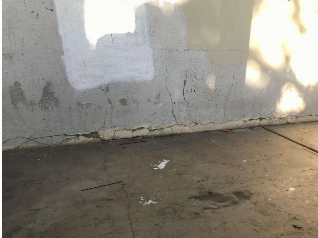
Figure 6: Plaster Cracking
