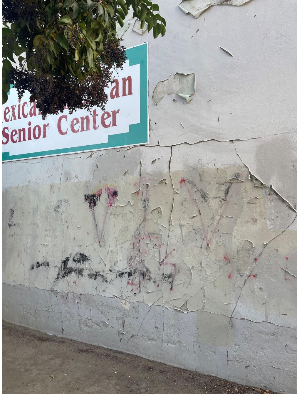
Figure 7: Plaster Cracking and Bowing Off Wall
