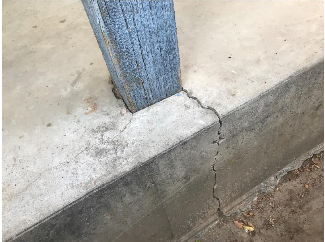
Figure 5: Dry Rot and Cracking at Base of Exterior Post
