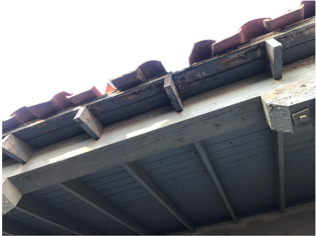
Figure 3: Water Damaged Straight Sheathing, Plywood Substrate, & Broken Roof Tiles
