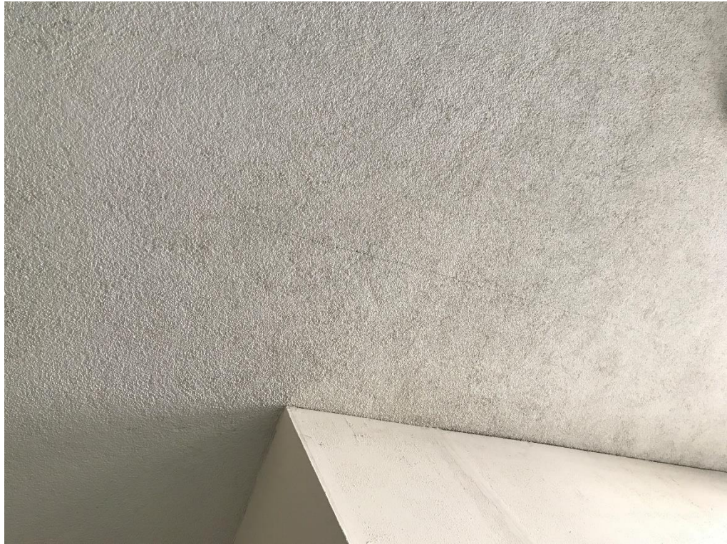
Figure 8: Cracking at Ceiling
