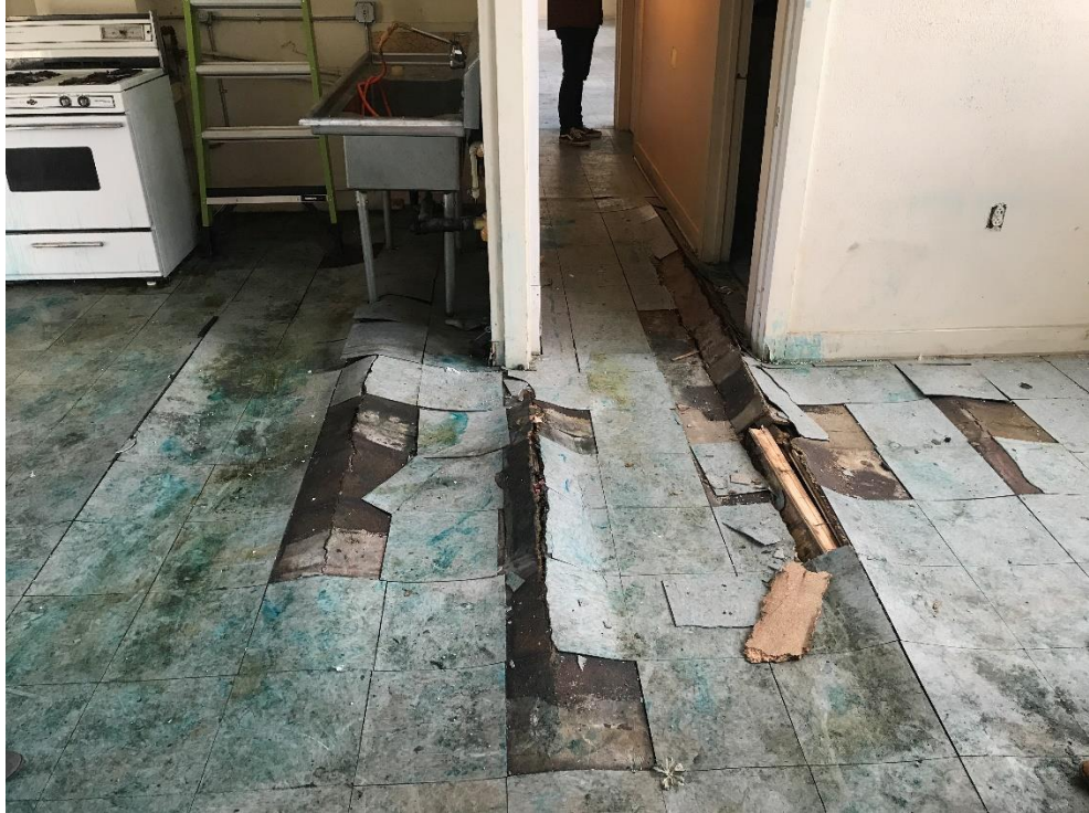
Figure 2: Water Damaged Floor Finish
