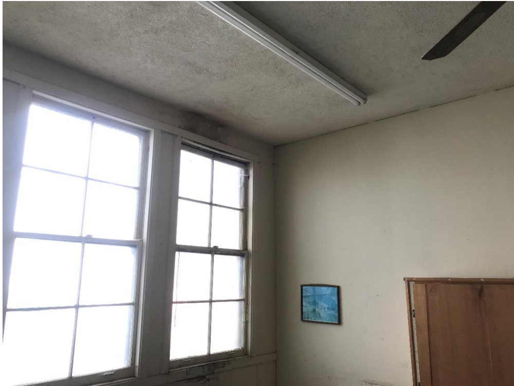
Figure 4: Water Damage Above and Below Window
