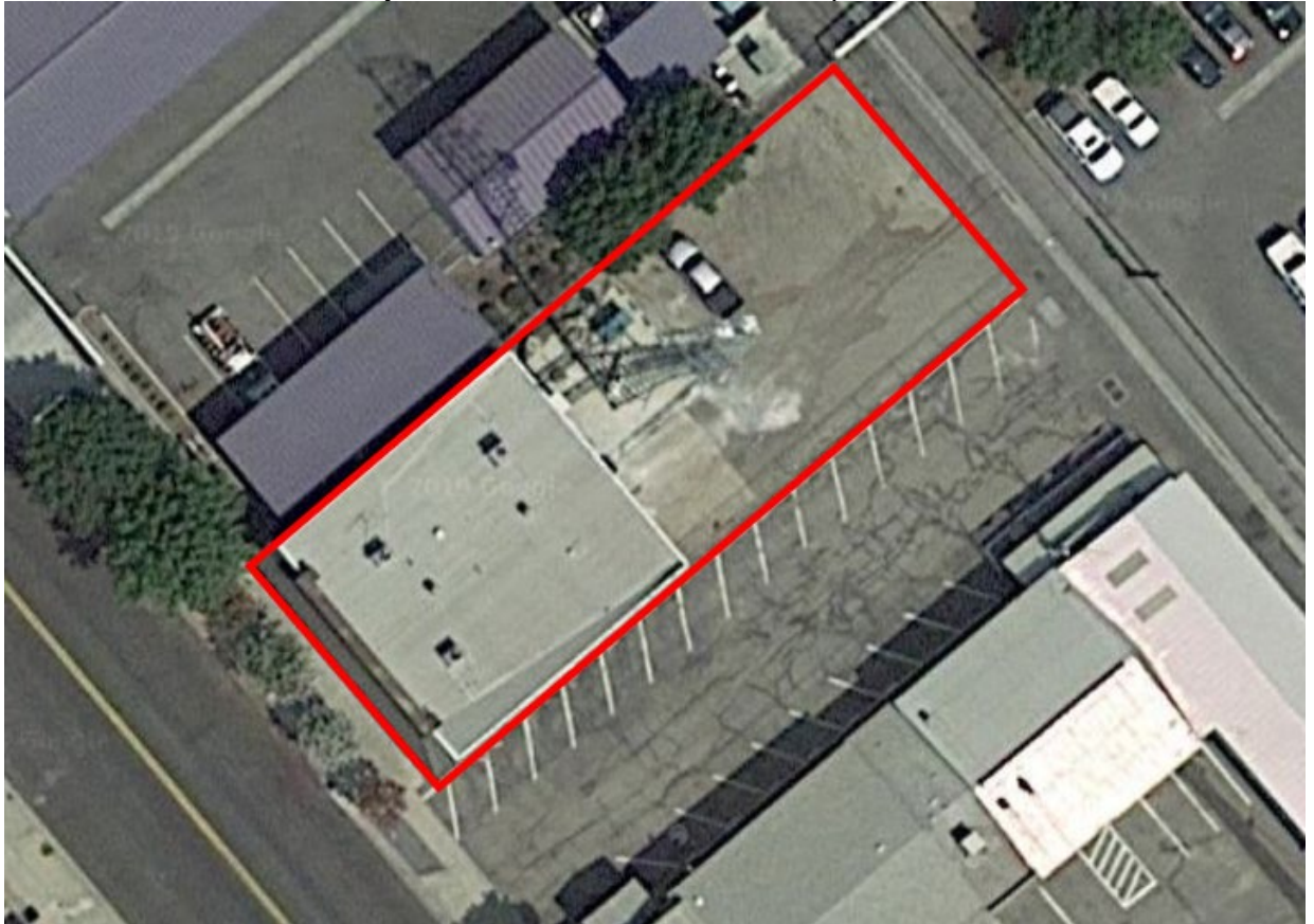
City of Madera – Madera Radio Dispatch site
