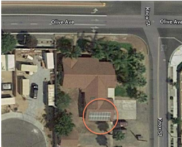
Picture 1. Solar Panels Before Theft
