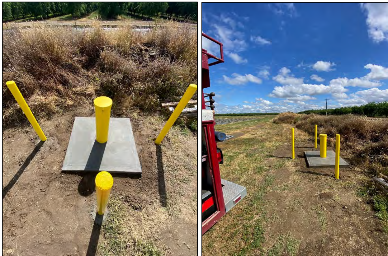
Figure 2: MW-5R Above Grade Completion
