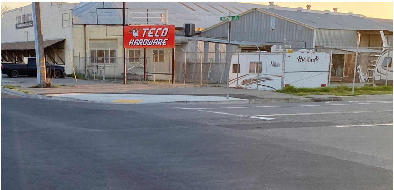
Figure 6 – Segment on Pine Street between Gil Avenue and West Almond (AFTER)
