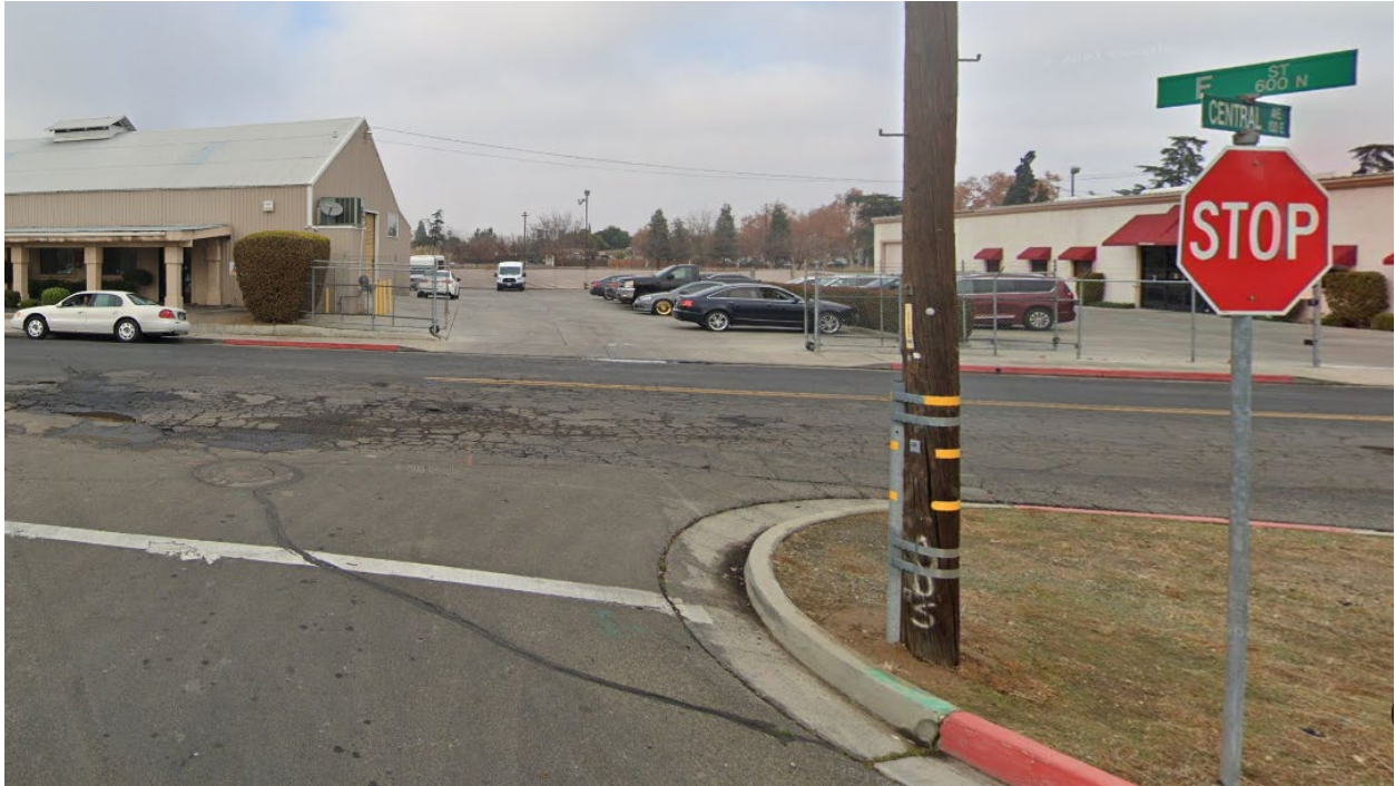
Figure 1 –Segment of Central Avenue between Gateway Drive and E Street (BEFORE)
