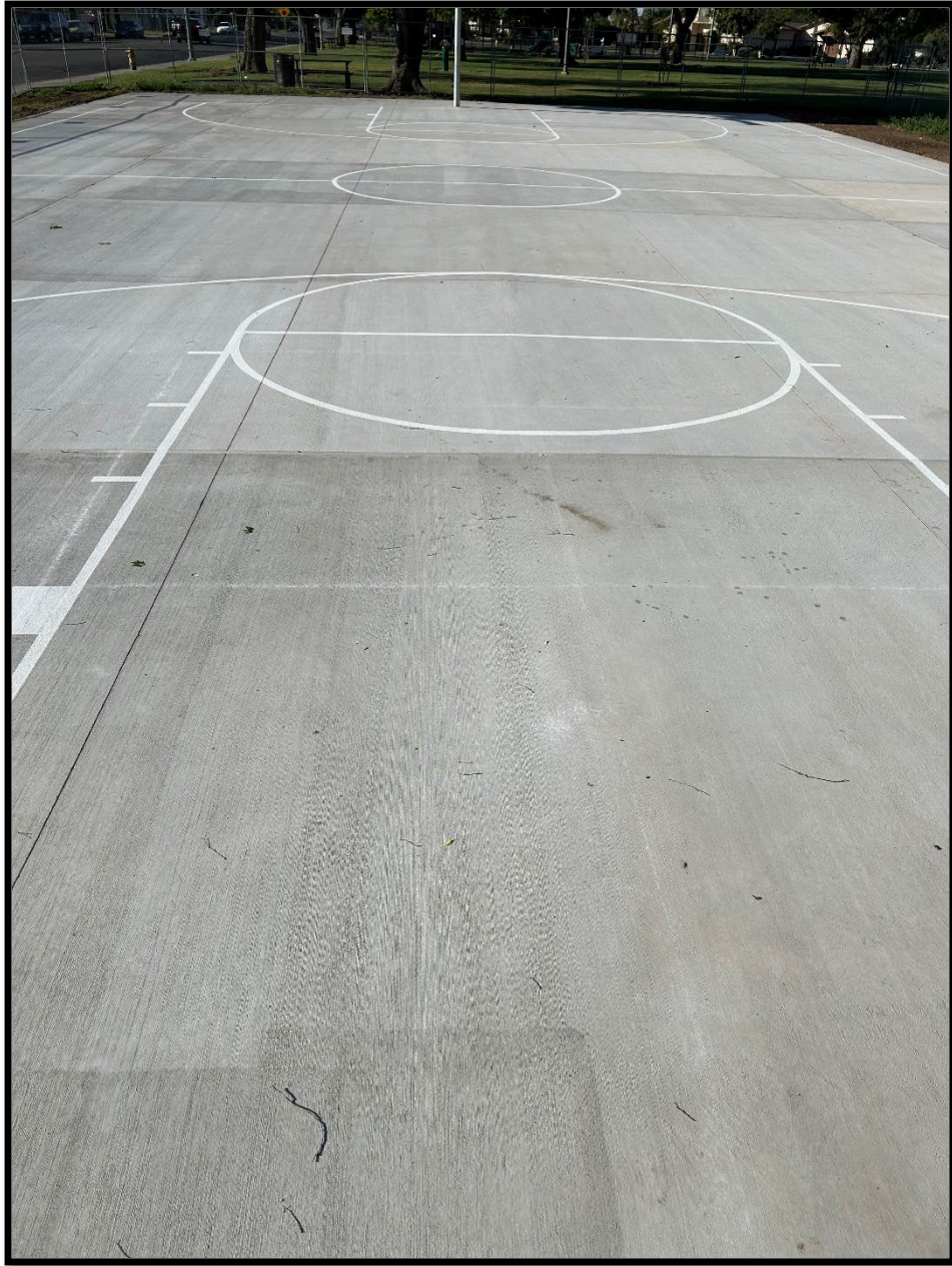
The Image Above Shows the Newly Reconstructed Basketball Courts at McNally Park.
