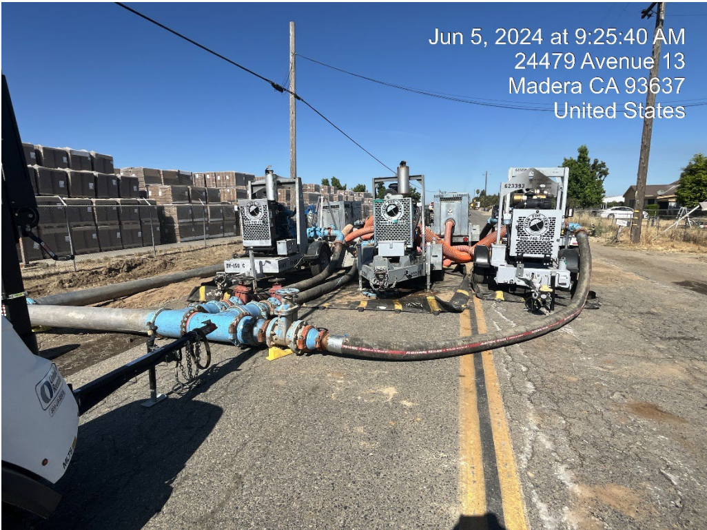
Bypass Pumping Set Up
