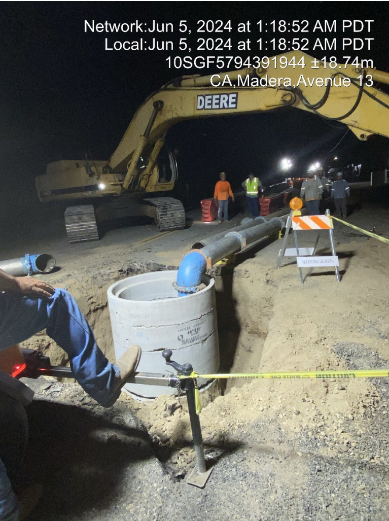
Bypass Pumping Set Up
