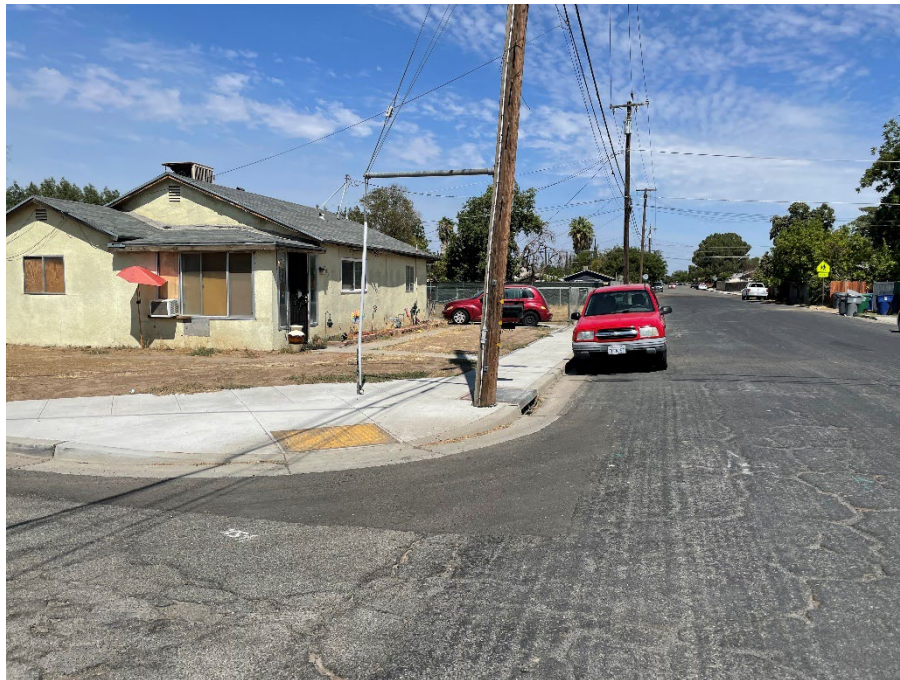
Figure 2 – After New Sidewalk along Maple Street
