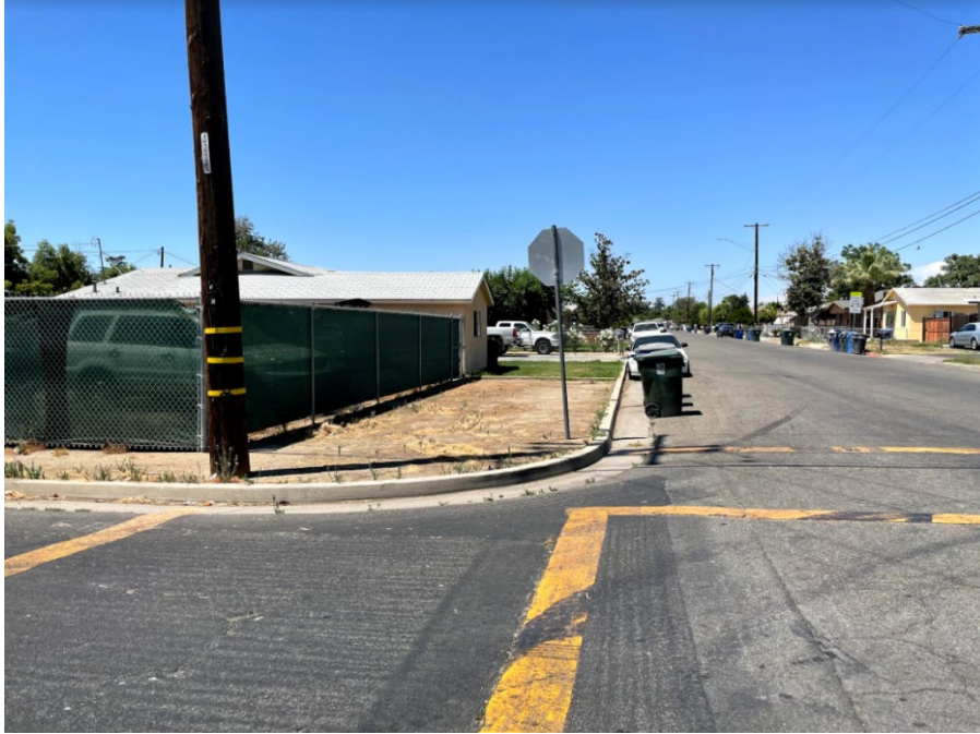
Figure 3 – Before New sidewalk along Santa Cruz Street
