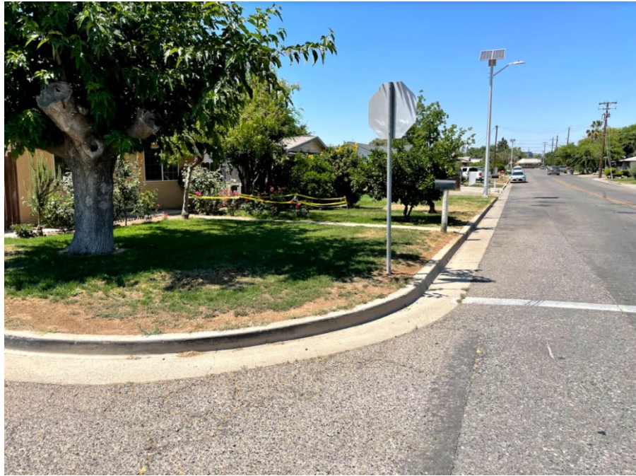
Figure 5 – Before New sidewalk along Monterey Street
