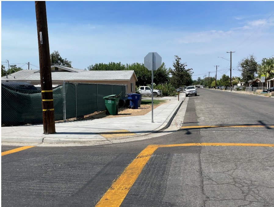
Figure 4 – After New sidewalk along Santa Cruz Street
