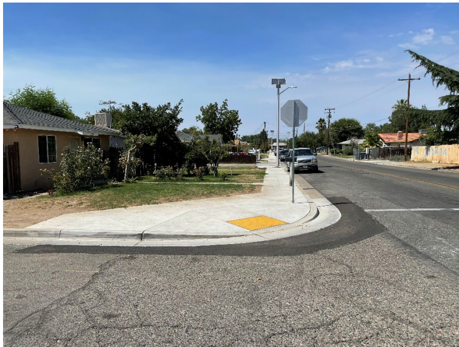
Figure 6 – After New sidewalk along Monterey Street
