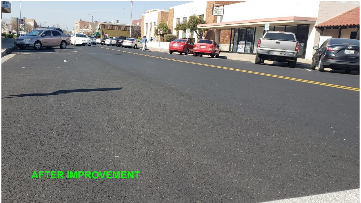
Figure 6 – D Street (After)
