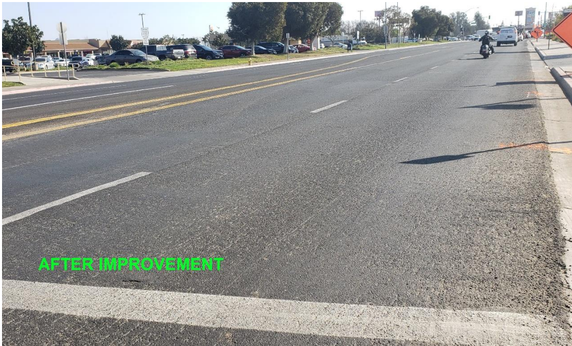
Figure 10 – Cleveland Avenue (After)
