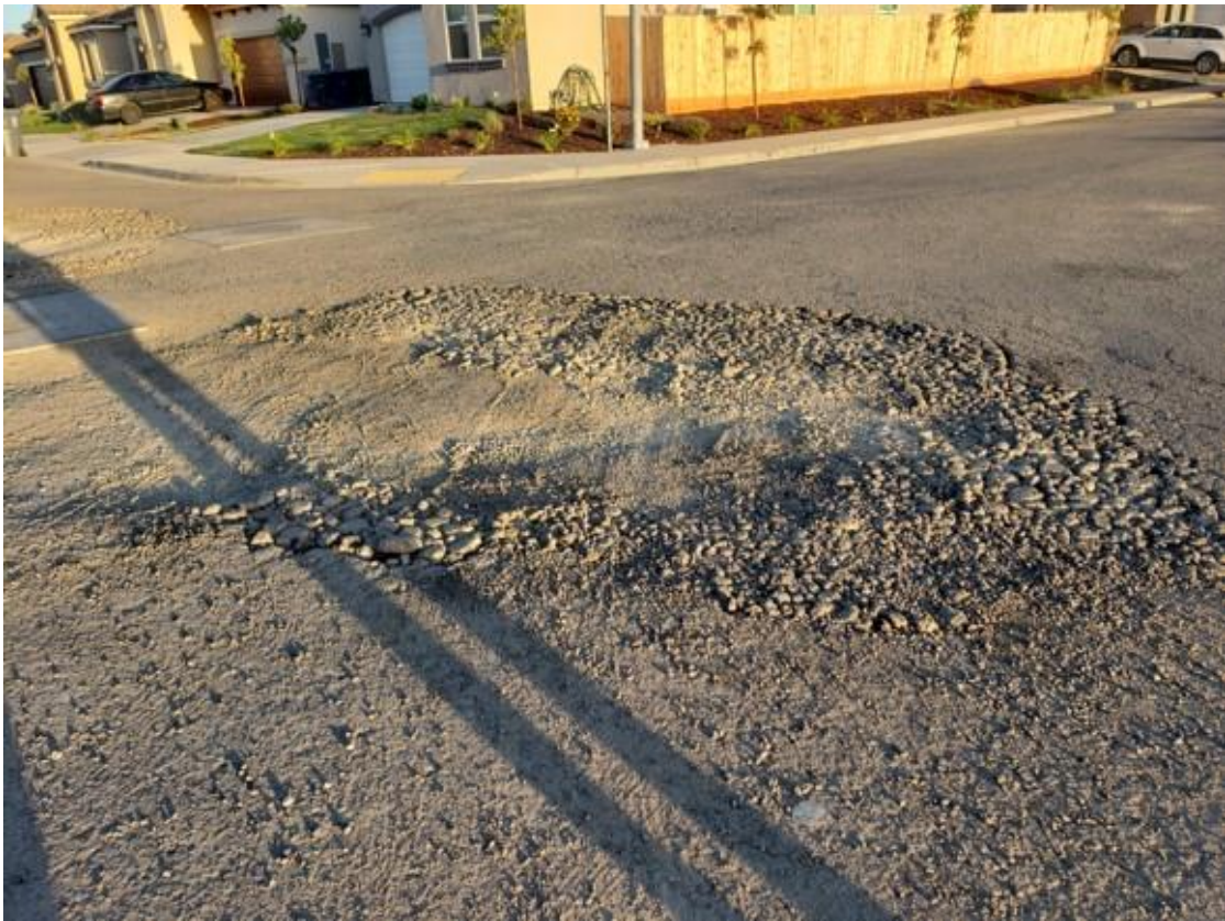
Figure 3 – Tierra Vista Subdivision (Before)
